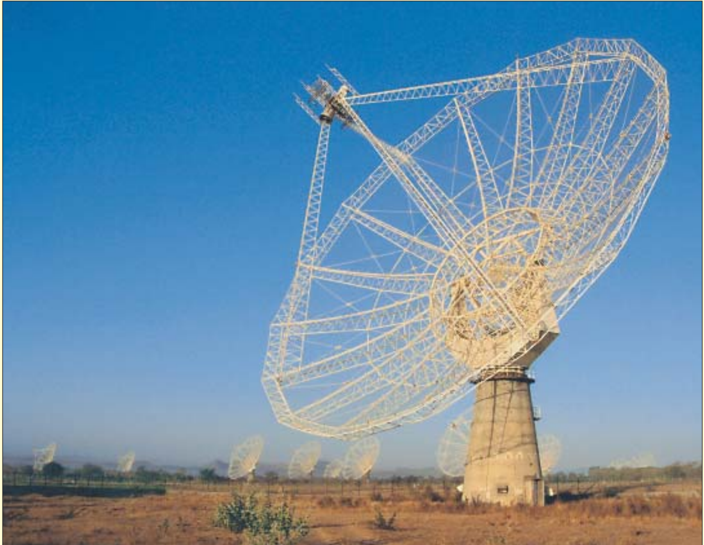
Giant Metre-wave Radio Telescope (GMRT) is the world's largest aperture synthesis radio telescope at metre wavelengths. It was commissioned at Khodad, about 80 km north of Pune in the year 1998
