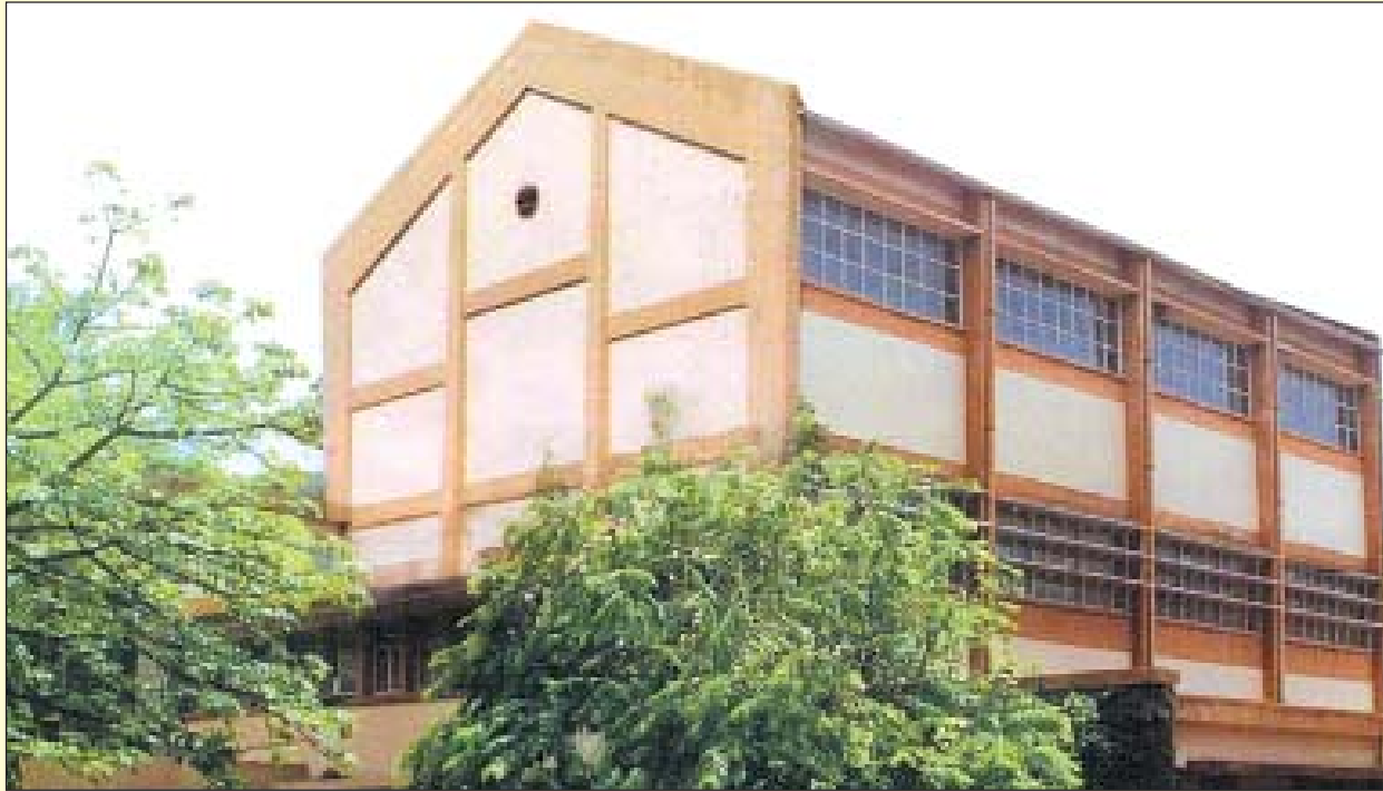
Apsara Reactor Building at Trombay
