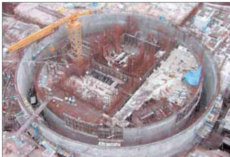
Construction in progress at RAPP-5 reactor building
