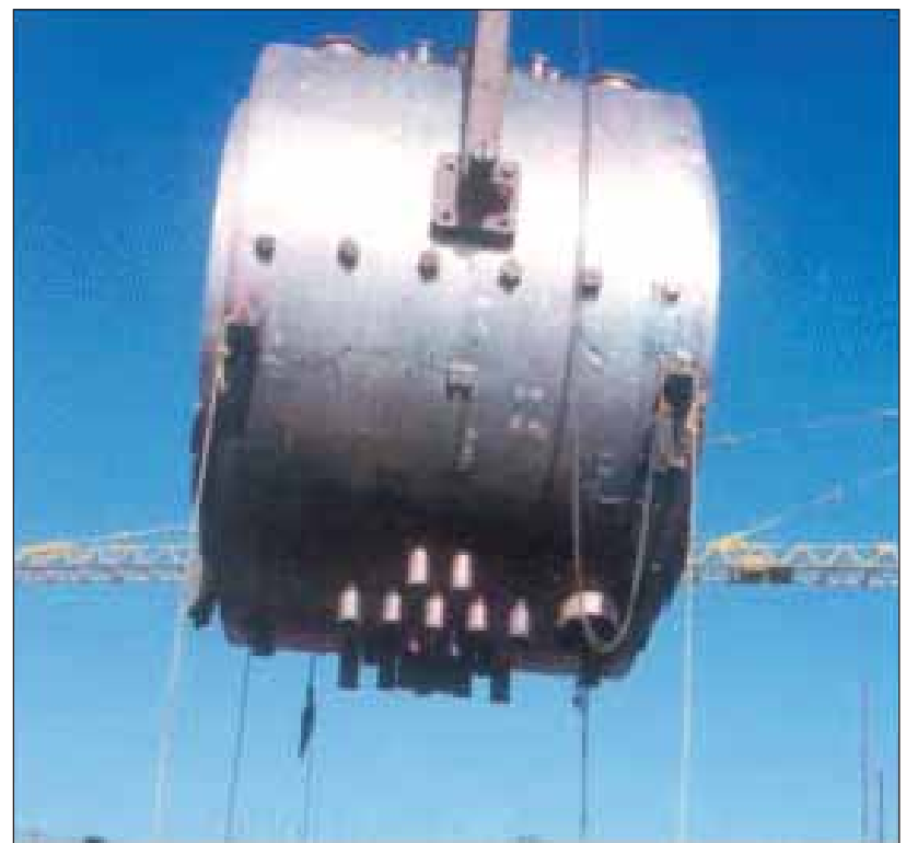
Calandria being lowered into reactor building
