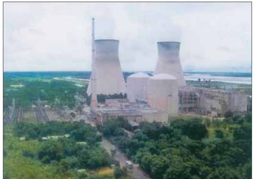
Narora Atomic Power Station
