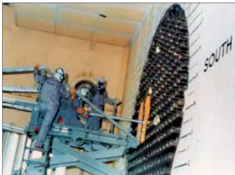
Coolant channel replacement operation
