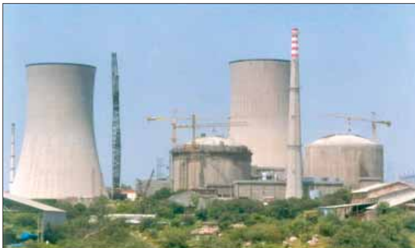
Rajasthan Atomic Power Station - 3 and 4 plants
