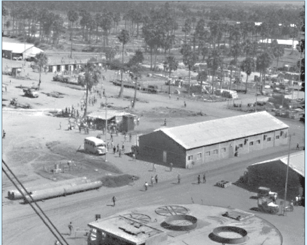
View of Tarapur construction site in 1964
