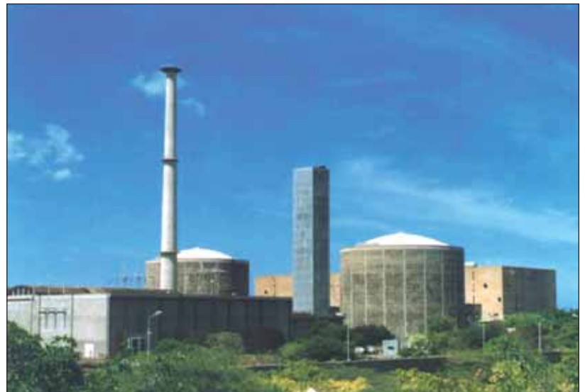
Madras Atomic Power Station
