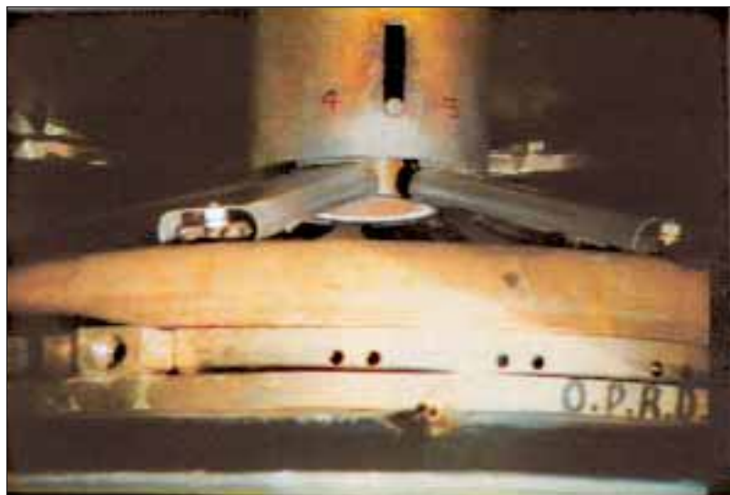
Over-pressure rupture disc repair at RAPS
