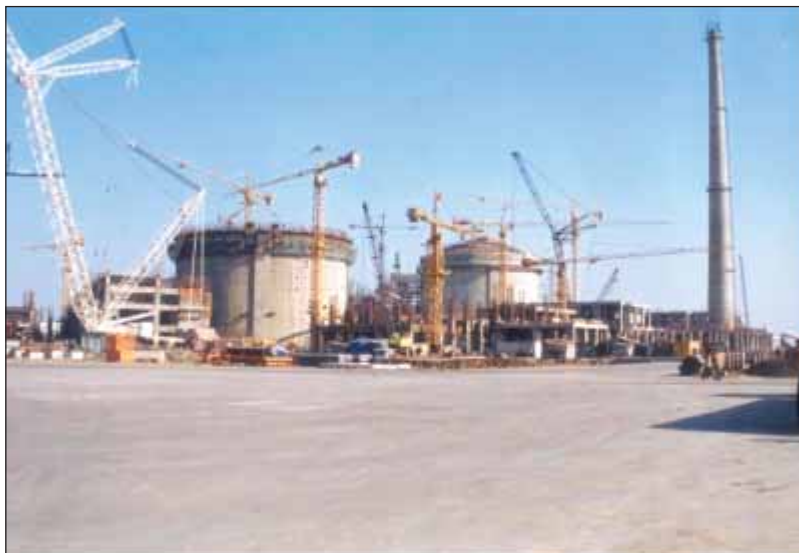
Construction work at Tarapur Units-3 and 4
