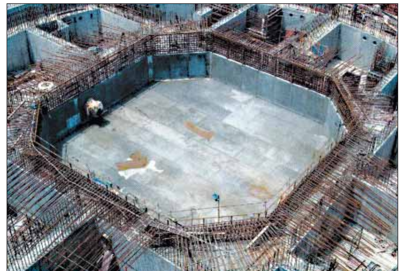
Concreting of core catcher in progress at Kudankulam
