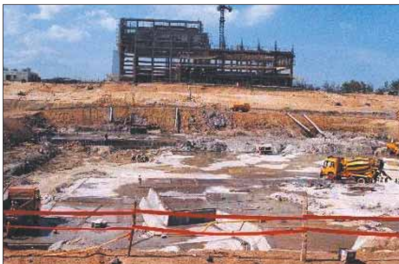
Excavation of nuclear island of FBR in progress at Kalpakkam
