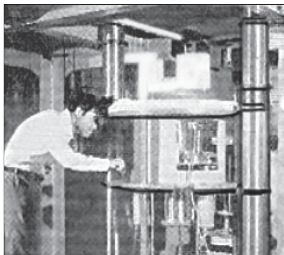
View of PURNIMA reactor
