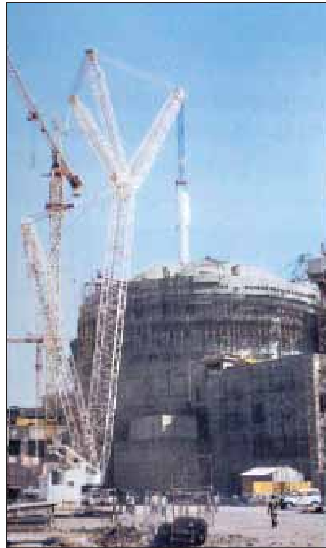
Lowering of steam generator into the containment building
