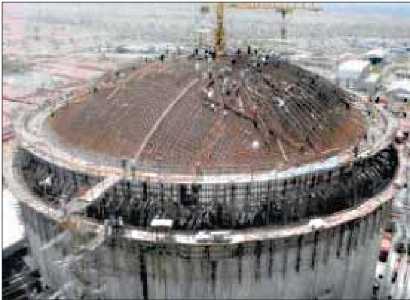
Re-engineered inner containment dome under construction
