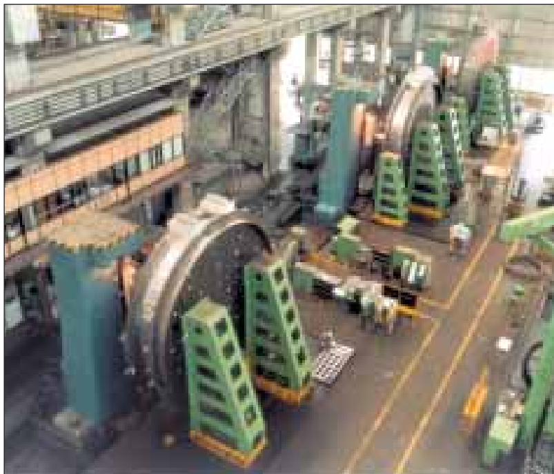
Machining of the end shields at manufacturer's works
