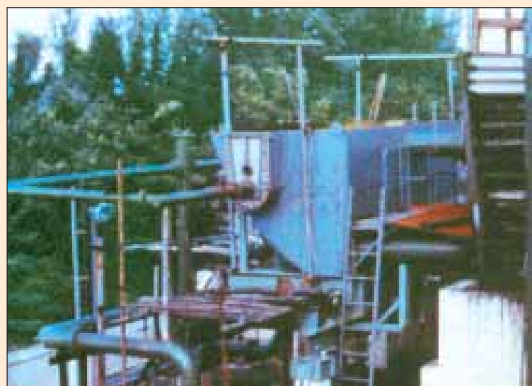
Sparger channel mock-up test facility at BARC
