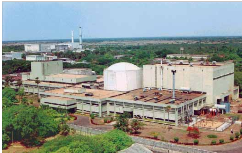
View of the FBTR complex at IGCAR
