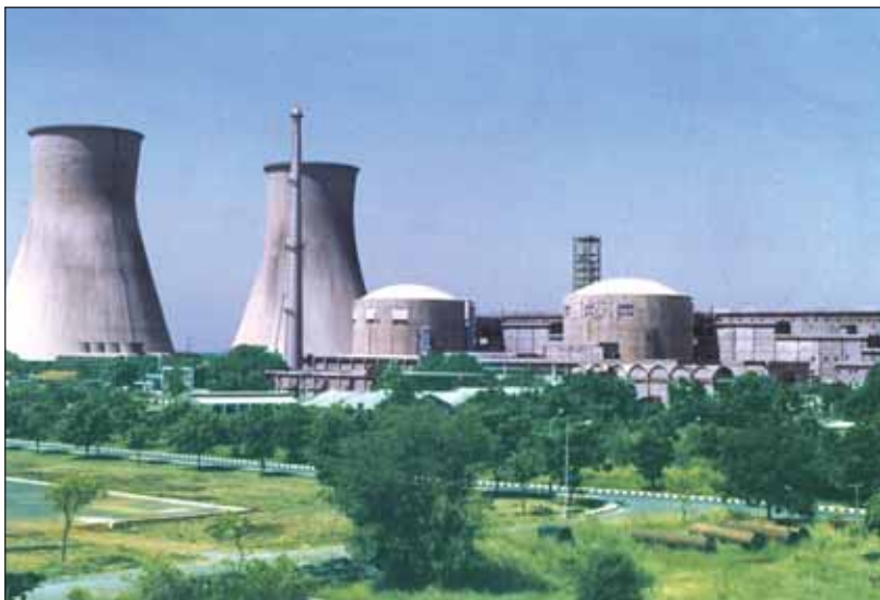
Kakrapar Atomic Power Station
