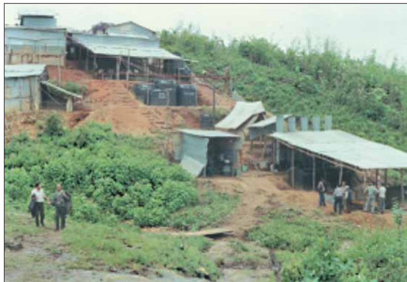
Uranium recovery pilot plant at Domiasiat, Meghalaya
