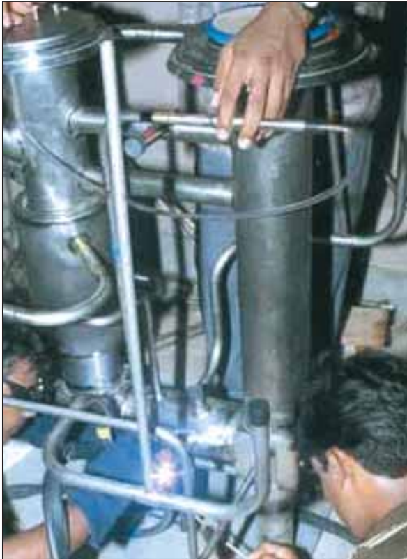
EODT dissolver under erection
