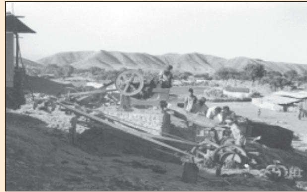
Ore recovery operation at Chhinjra
