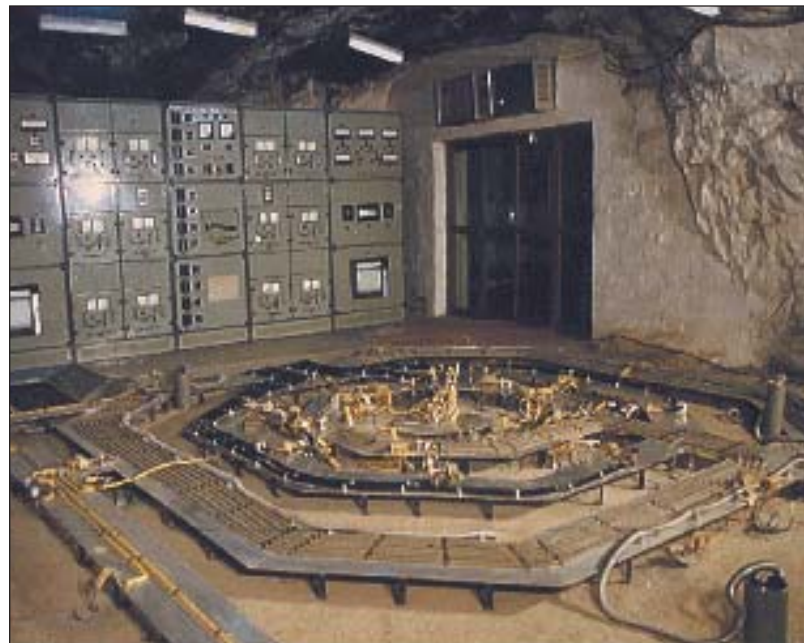
Thermo-mechanical experiment in underground chamber at Kolar Gold Fields
