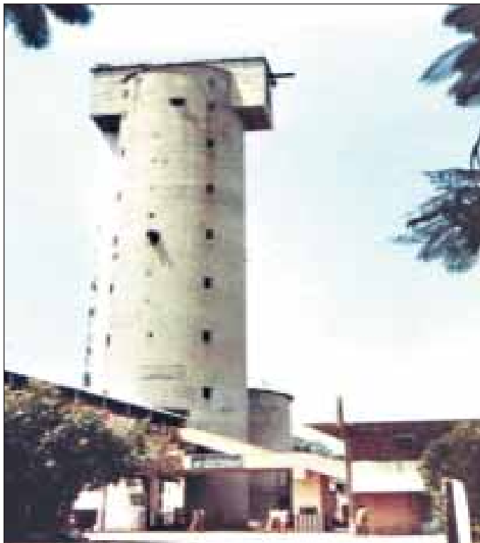
Uranium mine at Jaduguda
