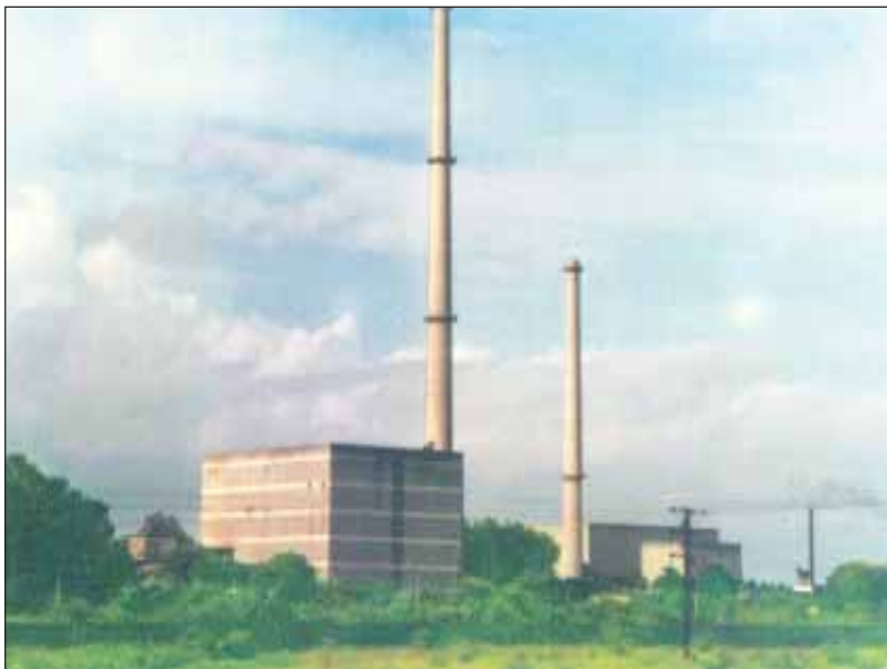
View of PREFRE plant at Tarapur
