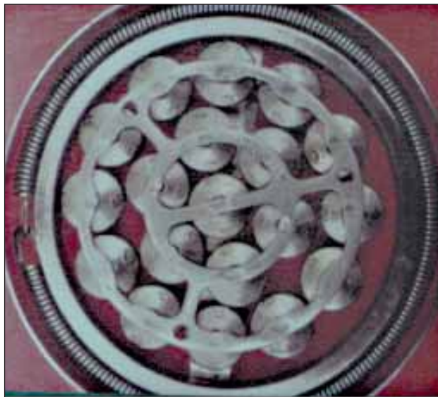
End view of coolant channel assembly of pressurized heavy water reactor.
