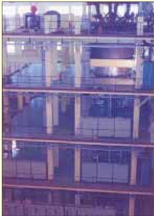
Large component test rig
