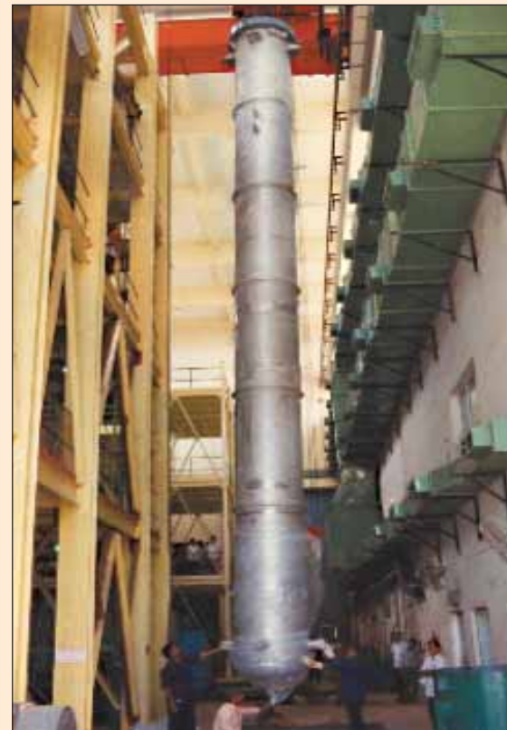
Sodium test vessel for CSRDM
