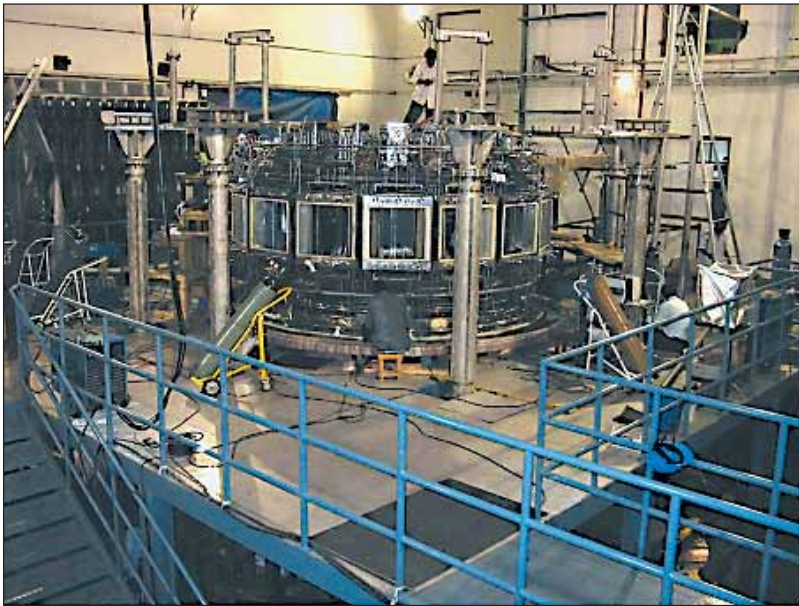
A view of SST-1 tokamak under erection & assembly at IPR
