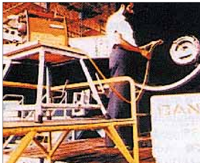
Isotope radiography testing of an aircraft engine
