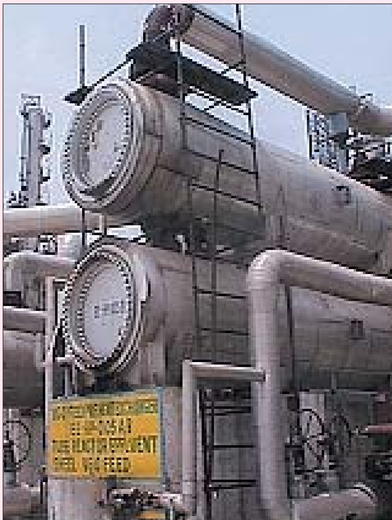
Radiotracer experiment for leak location in heat exchangers
