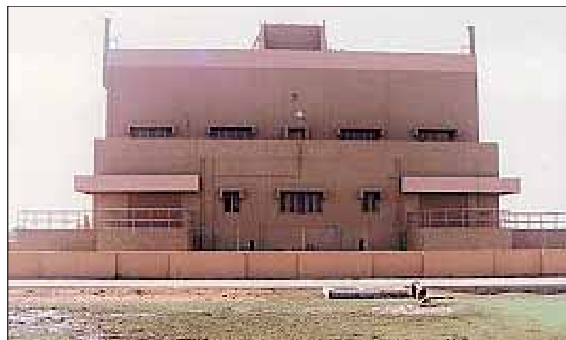
Sewage Sludge Hygienisation Research Irradiator (SHRI) Facility at Vadodra, Gujarat
