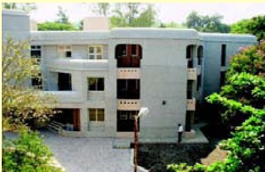
Girls' Hostel for National Centre for Cell Science (NCCS) Pune
