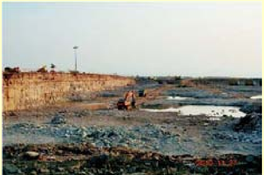
Excavation work in progress at RAPP-7&8
