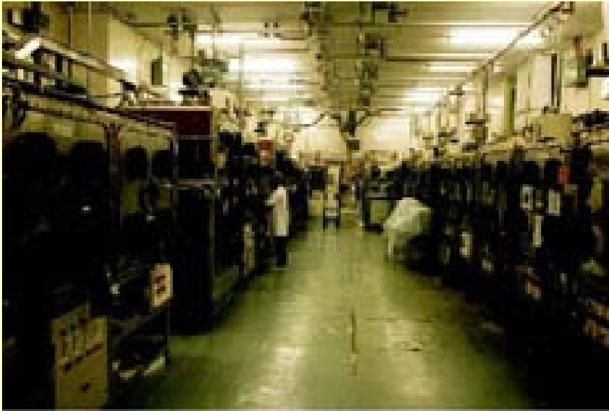
New fabrication line of Advanced Fuel Fabrication Facility for PFBR
