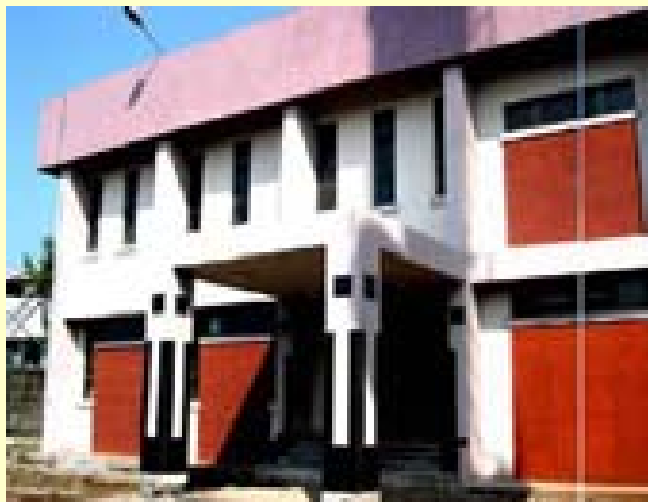
Integrated Facility for Radiation Technology
