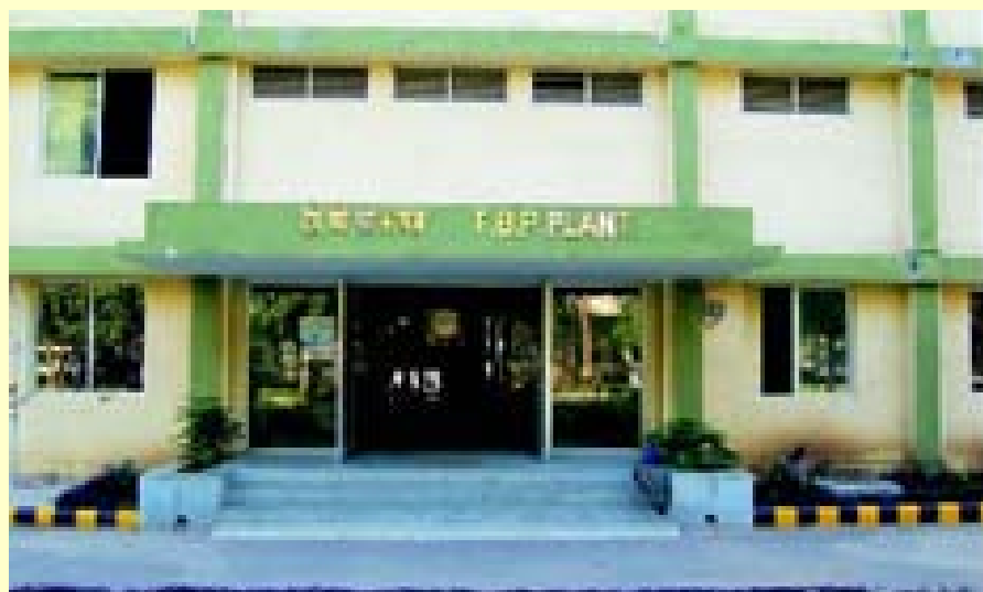
TBP plant at Heavy Water Plant, Baroda
