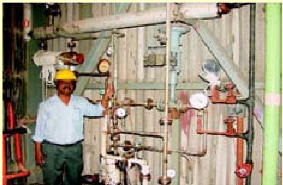
View of the Oxygen-18 column top condensers at Heavy Water Plant, Tuticorin
