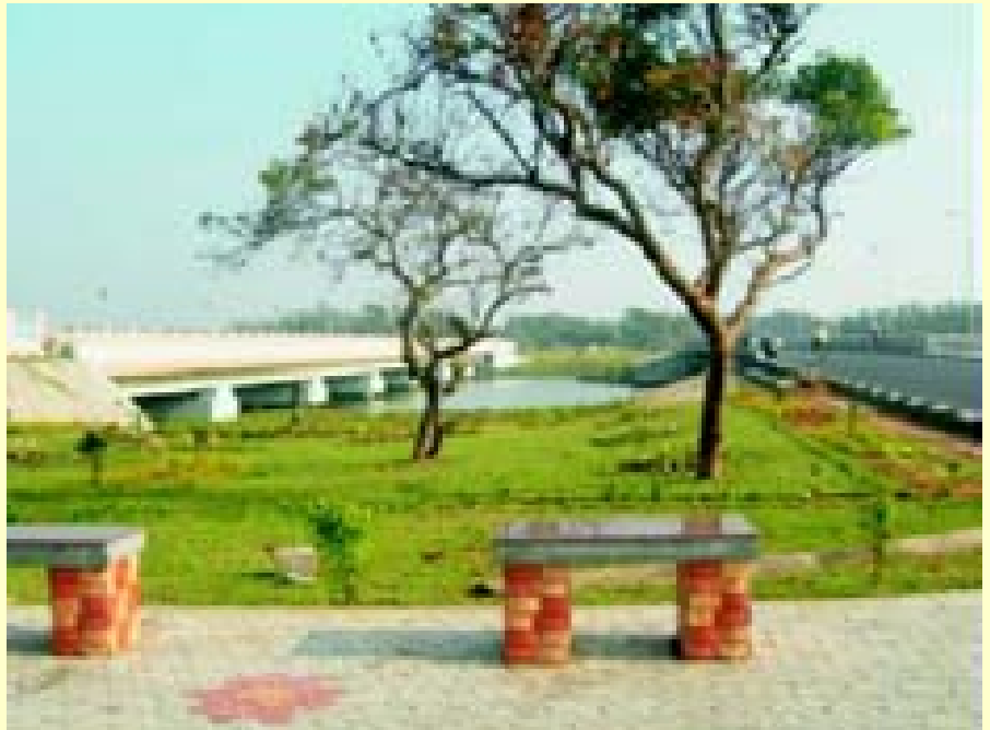
Development works in between bridges
