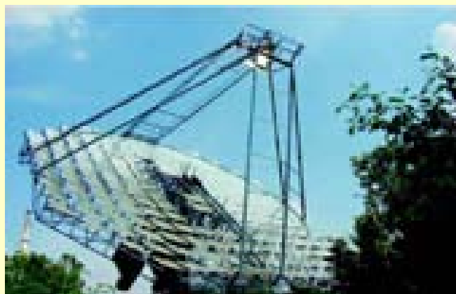
Solar Evaporator for steam generation at the Heavy Water Plant, Kota
