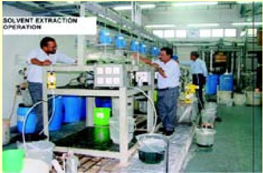
Operation of Mixer Settler in Solvent Extraction Facility at Heavy Water Plant, Tuticorin
