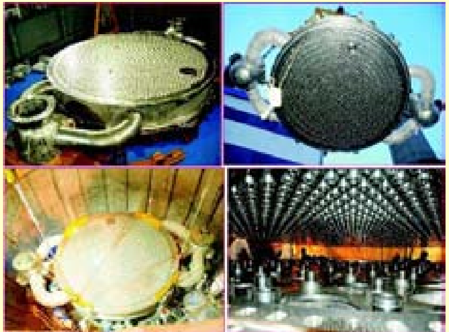
Grid Plate erection
