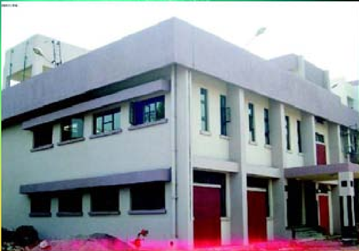
Integrated Facility for Radiation Technology Building at Vashi, Navi Mumbai
