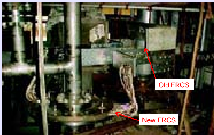
Parallel Channel as installed in ITL
