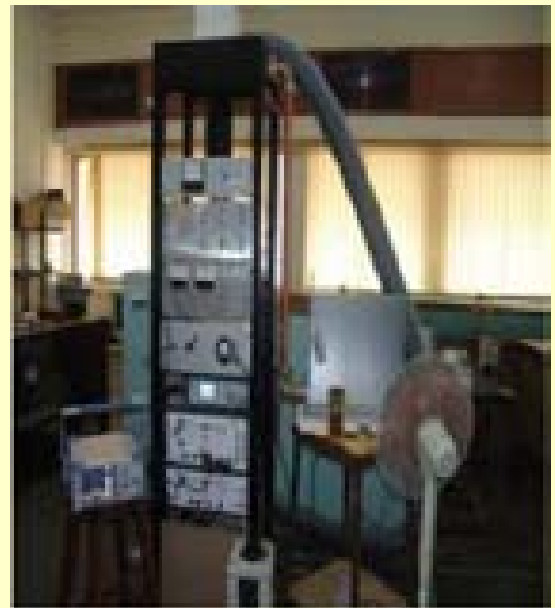
3 kW @ 350 MHz Driver for RF system
