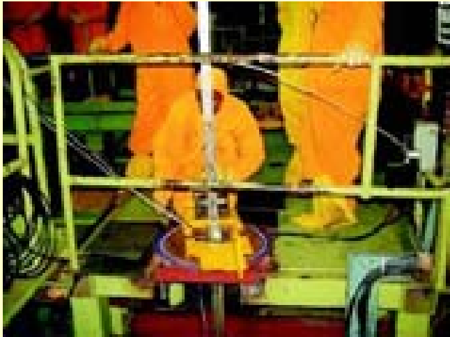
In-core repair work in the Calandria Vault of KAPS-1
