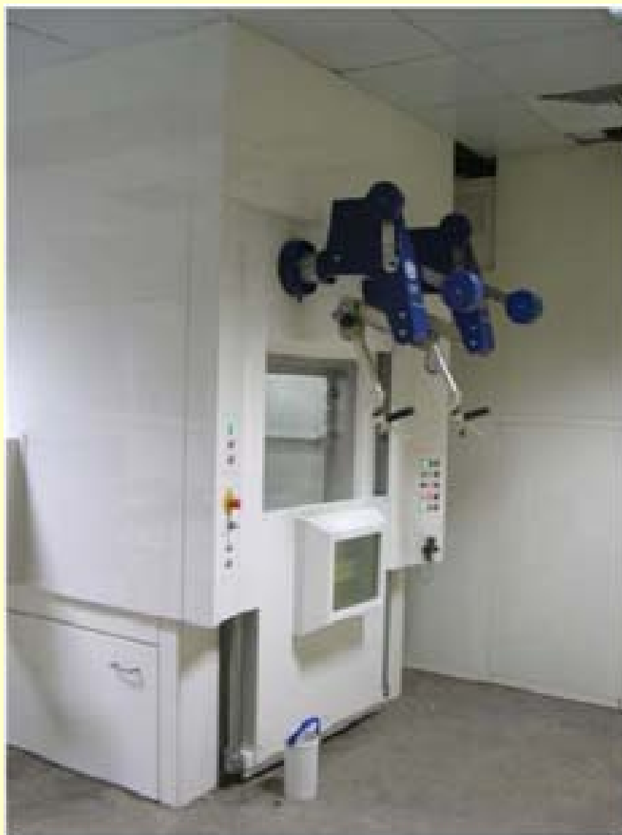
Molybdenum-99 Column Generator Plant
