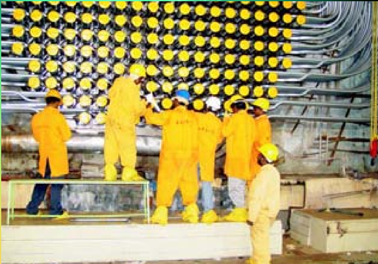
Enmasse Coolant Channel Replacement in action
