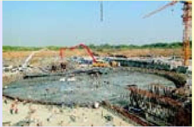
First Pour of Concrete in progress at KAPP-3&4
