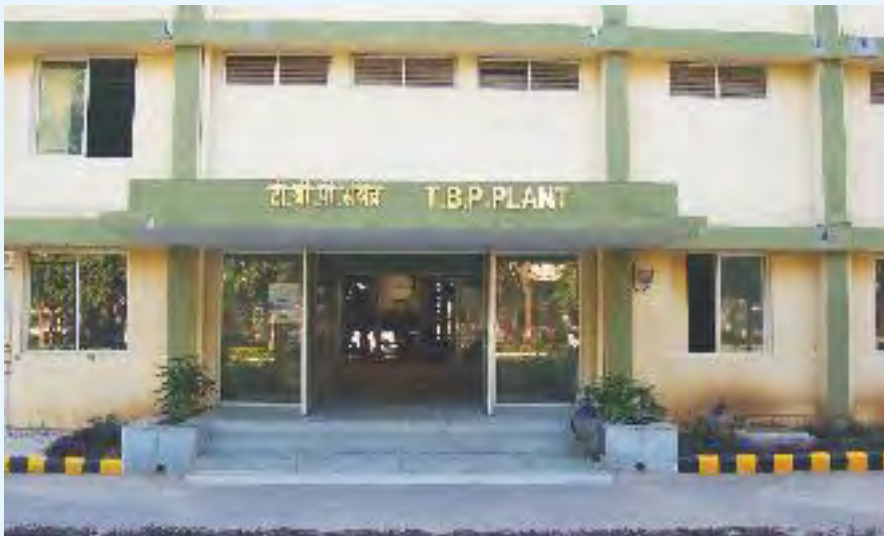
TBP plant at Heavy Water Plant, Baroda
