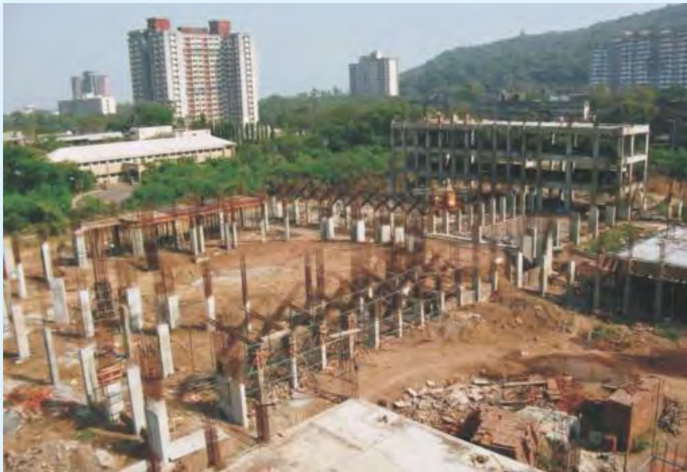
Under construction : Convention Centre at Anushaktinagar
