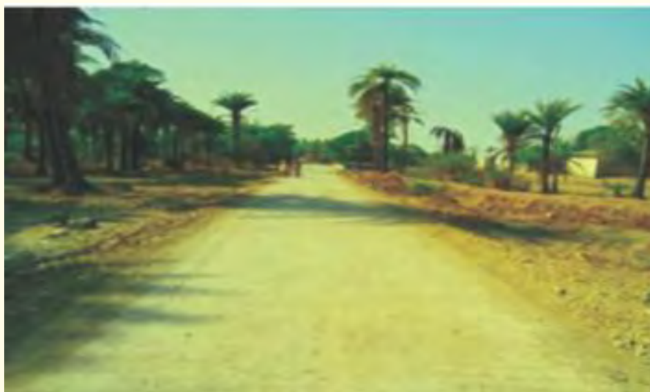
Construction of approach road to Ghivali
