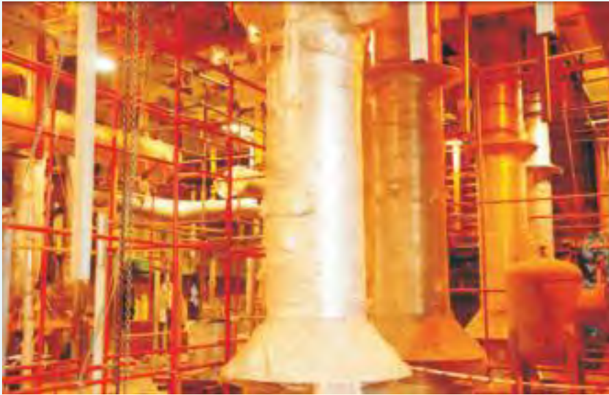
Steam generator erection
