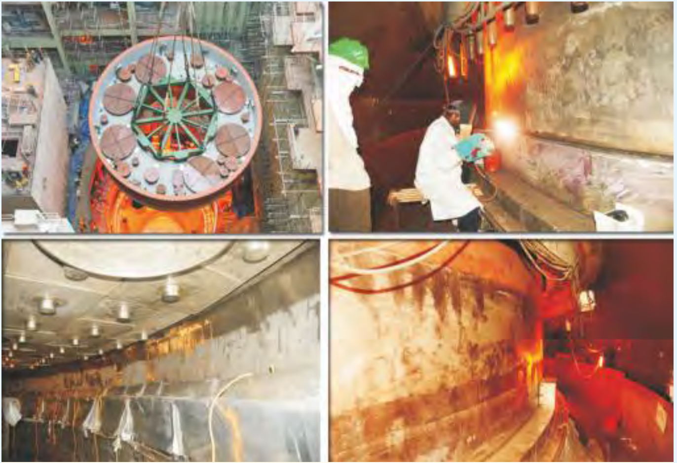
Roof slab erection & Integration with Main Vessel
