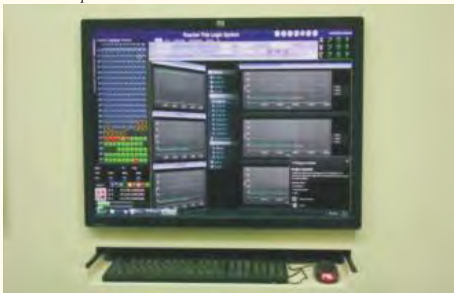
Operator Console for Trombay-PLC-based Reactor Trip Logic System & Alarm Annunciator
