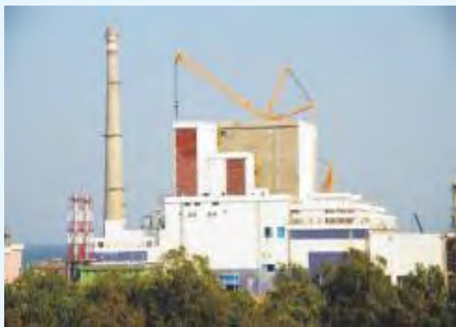
Nuclear Island Connected Buildings (NICB) of PFBR
