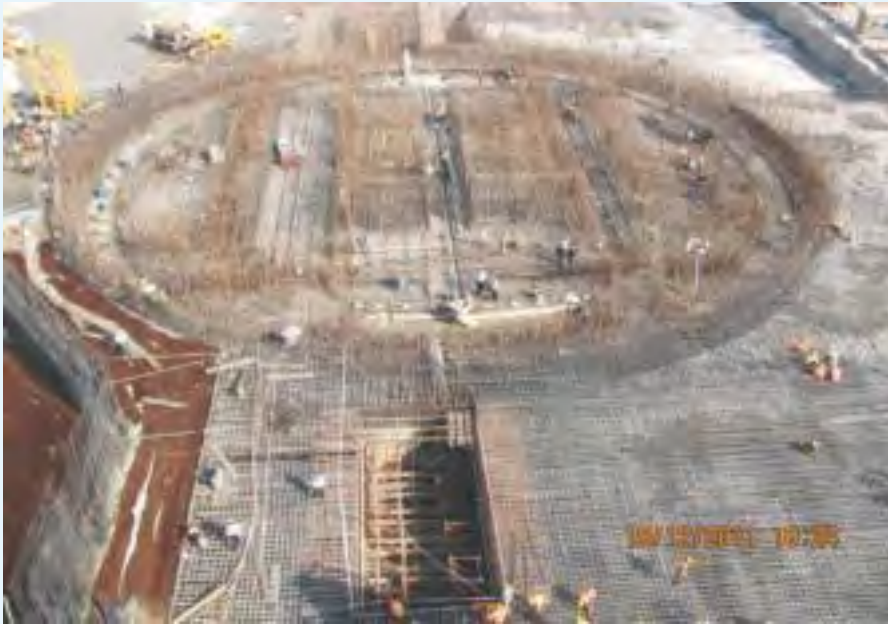
View of the Nuclear Building-7 of the Rajasthan Atomic Power Project-7&8
