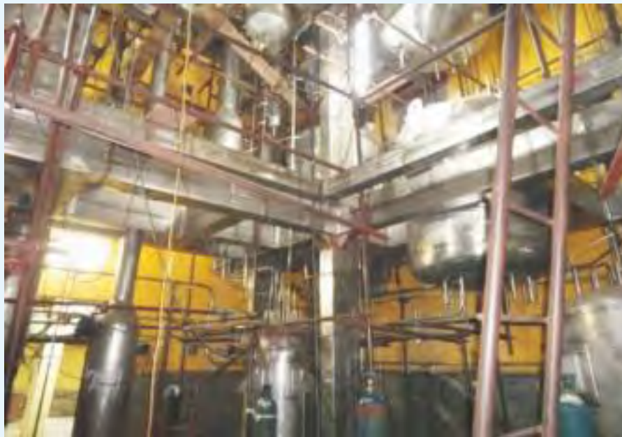
P3A project - Incell process piping in progress
