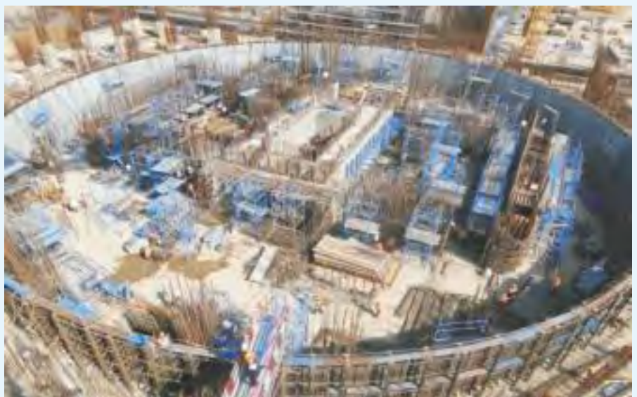
Internal view of Reactor Building-3, KAPP-3&4
