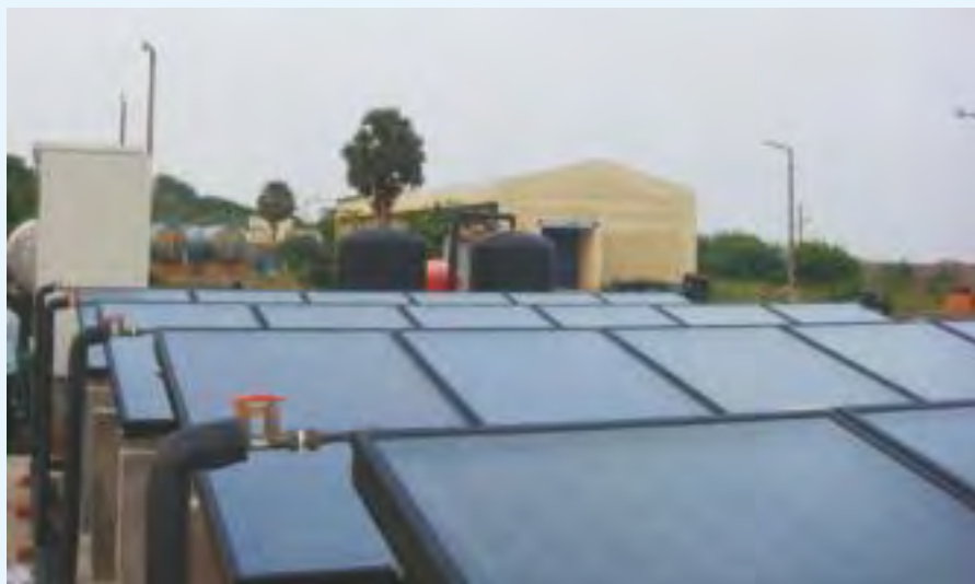
Solar driven 1000 litres/day Multi-Effect Humidification facility at Kalpakkam
