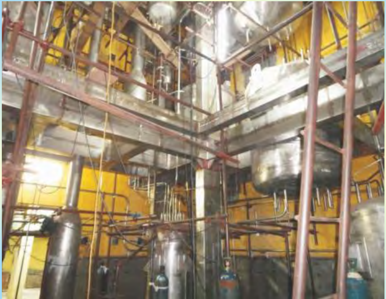
P3A project- Incell process piping work under progress
