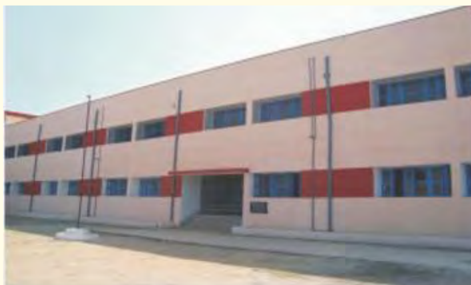
Construction of Rooms & Labs for Science wing of the State Govt. (Girls) Sr.Hr. Sec. School at Rawatbhata, Rajasthan
