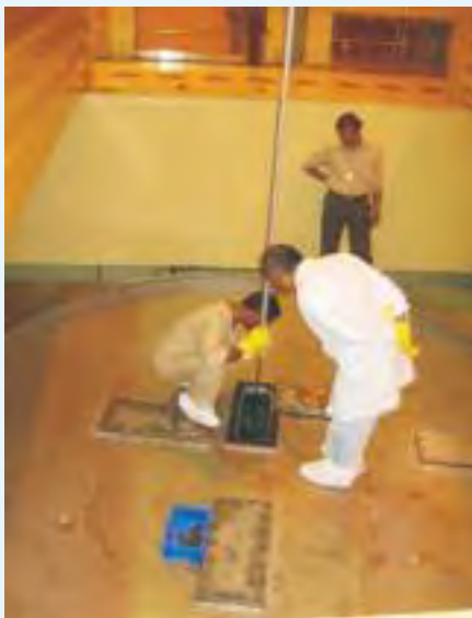
Installation of flux mapping assembly around central core location
