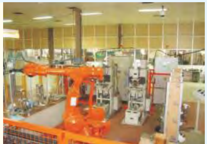
Robot integrated with two end-plate welding machines
