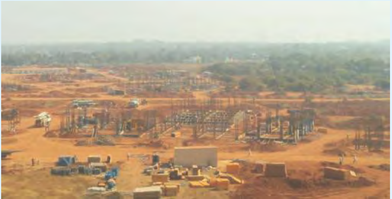
Fast Reactor Fuel Cycle Facility Project
