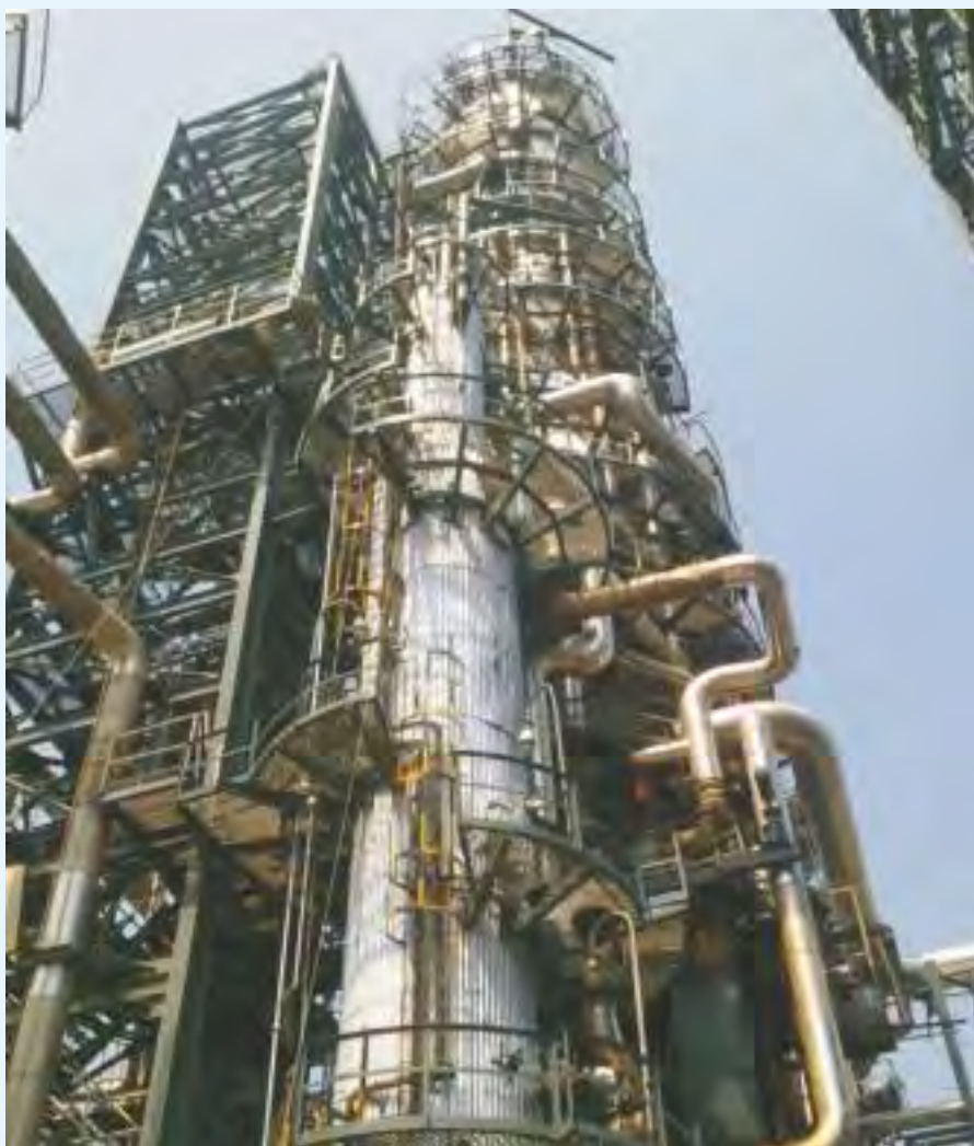
Gamma Scanning of a Process column
