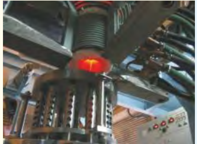
Remote cutting of Joule melter side electrodes
