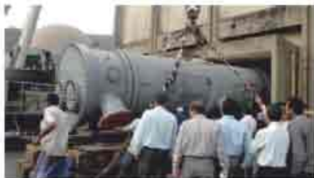
Process-water/Seawater heat exchanger replacement
