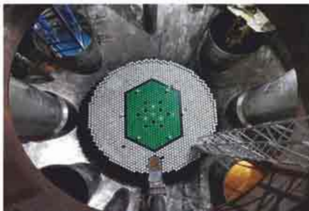
Inside view of reactor vessel with Sub-assemblies loaded, BHAVINI
