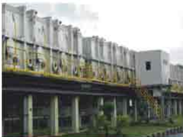
Multi-Stage Flash (MSF) section of NDDP Kalpakkam
