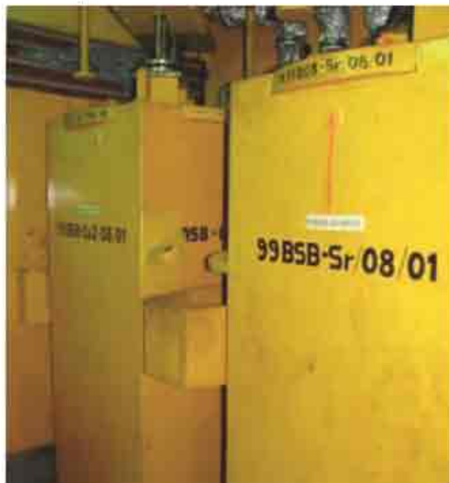
Facility for treatment of ILW a) Self-shielded ion exchange columns.
