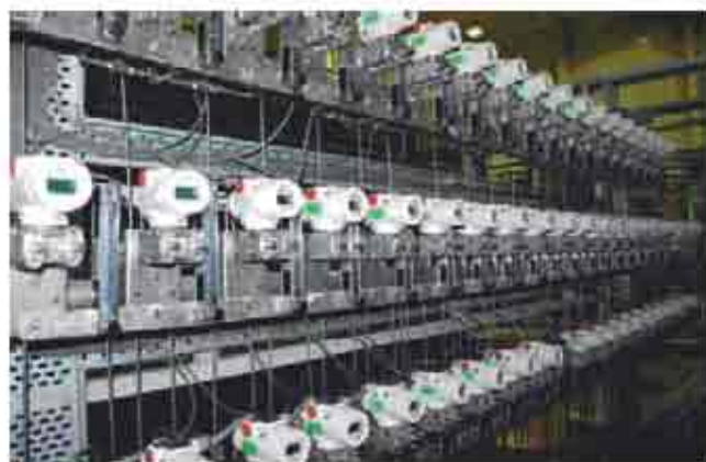
A view of the transmitter gallery for the C&I of DFRP
