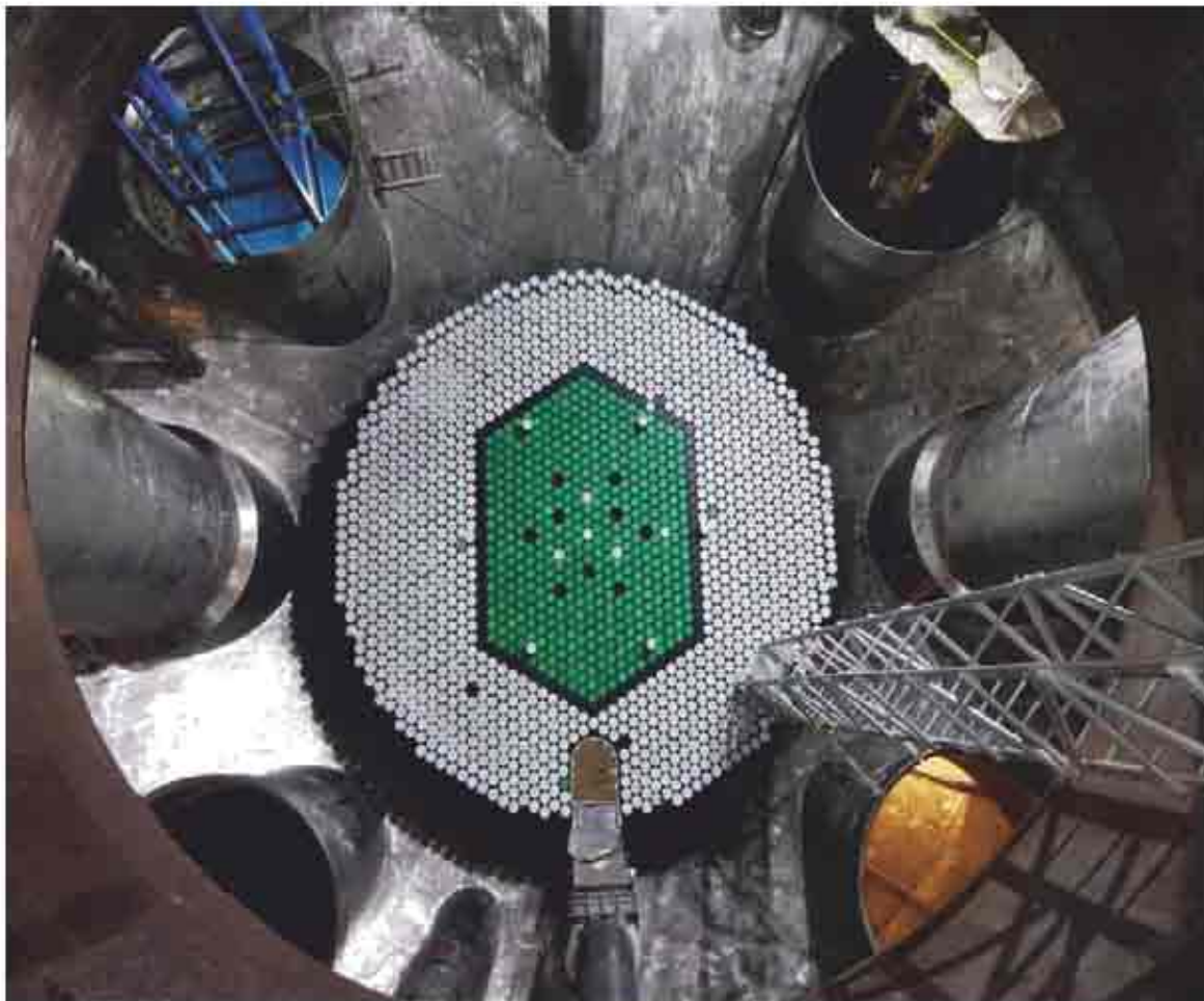
Inside view of PFBR reactor vessel with loaded Sub-assemblies
