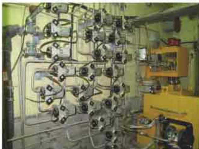
b) Ion exchange feed pump with associated valving
