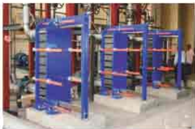
Klystron Cooling System Heat Exchangers
