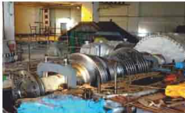
Erection of Turbine IP rotor
