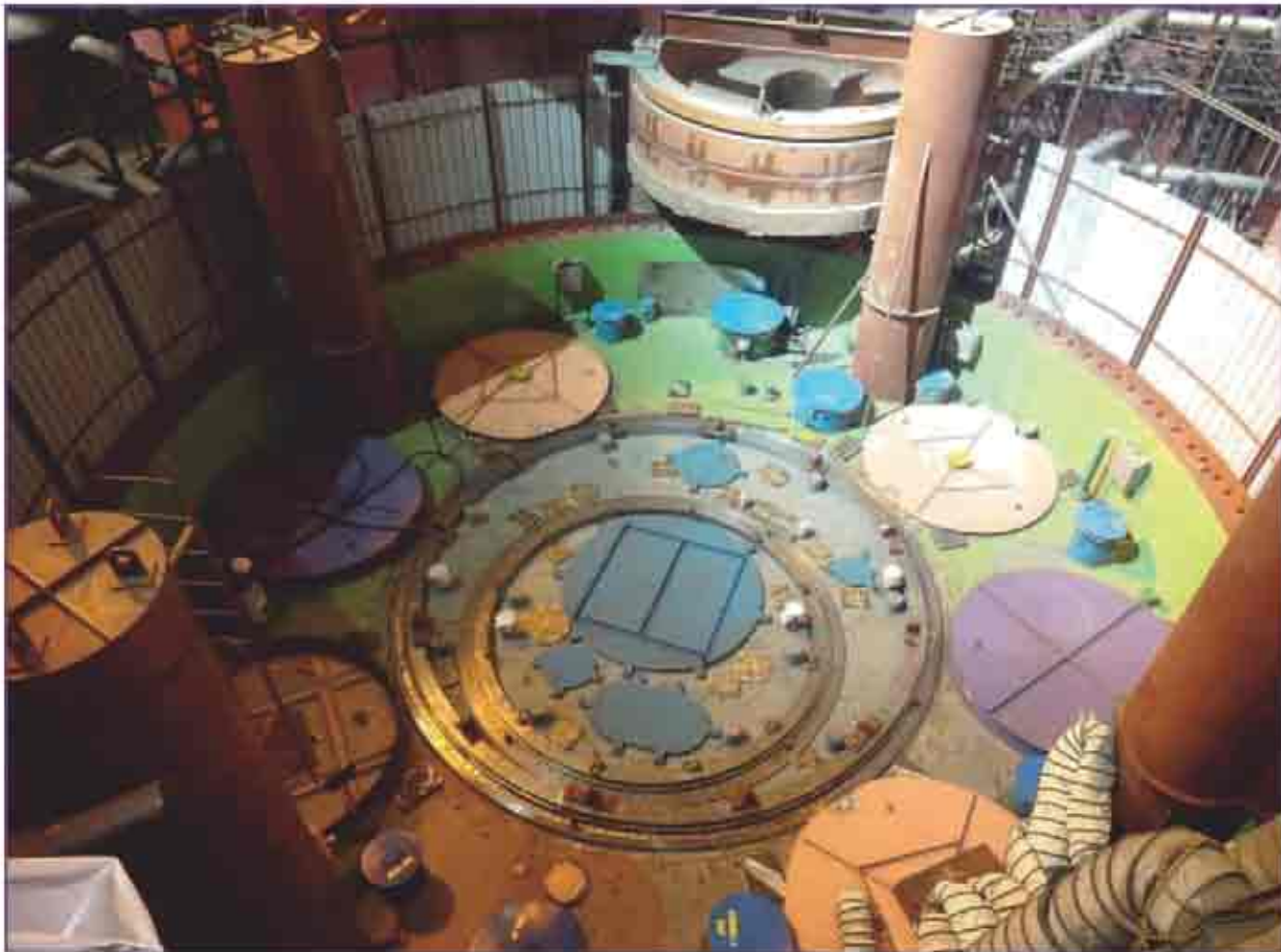
Top view of PFBR reactor vault with rotatable plugs in position
