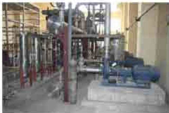
Klystron Cooling System Piping
