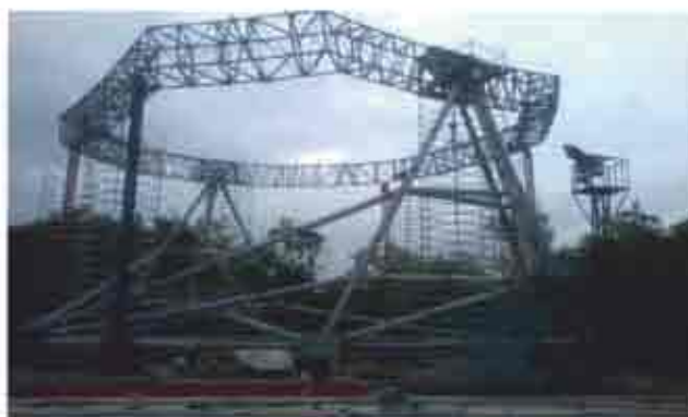
Assembly of MACE telescope at Hyderabad
