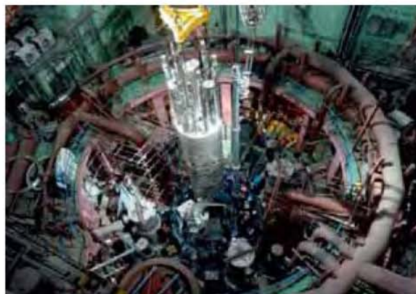
Erection of control plug
