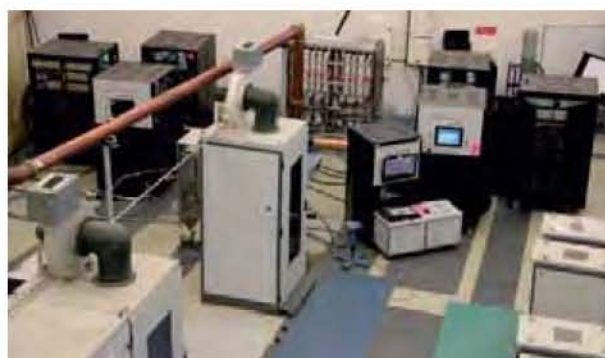
High power solid state amplifier stations installed in Indus-2 RF area
