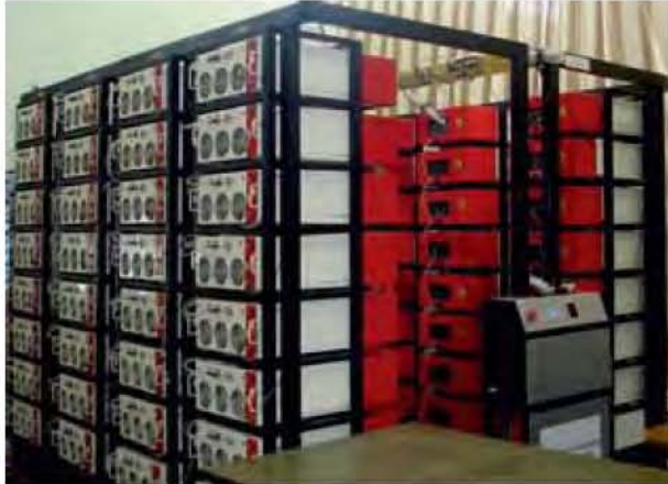
36 kV, 24 Amp DC power supply
