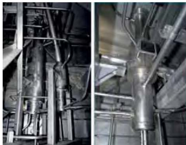
View of the dissolver and electrolyser along with the associated piping system
