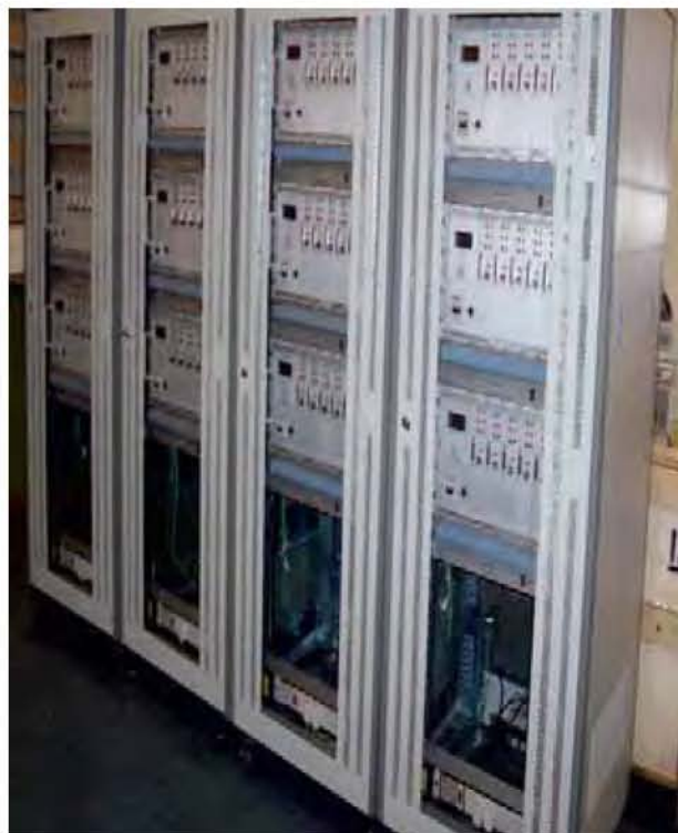
Power supply for IRFEL beamline magnets
