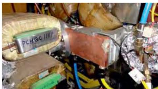
Cooling arrangement in Indus-2 dipole chamber's end plate
