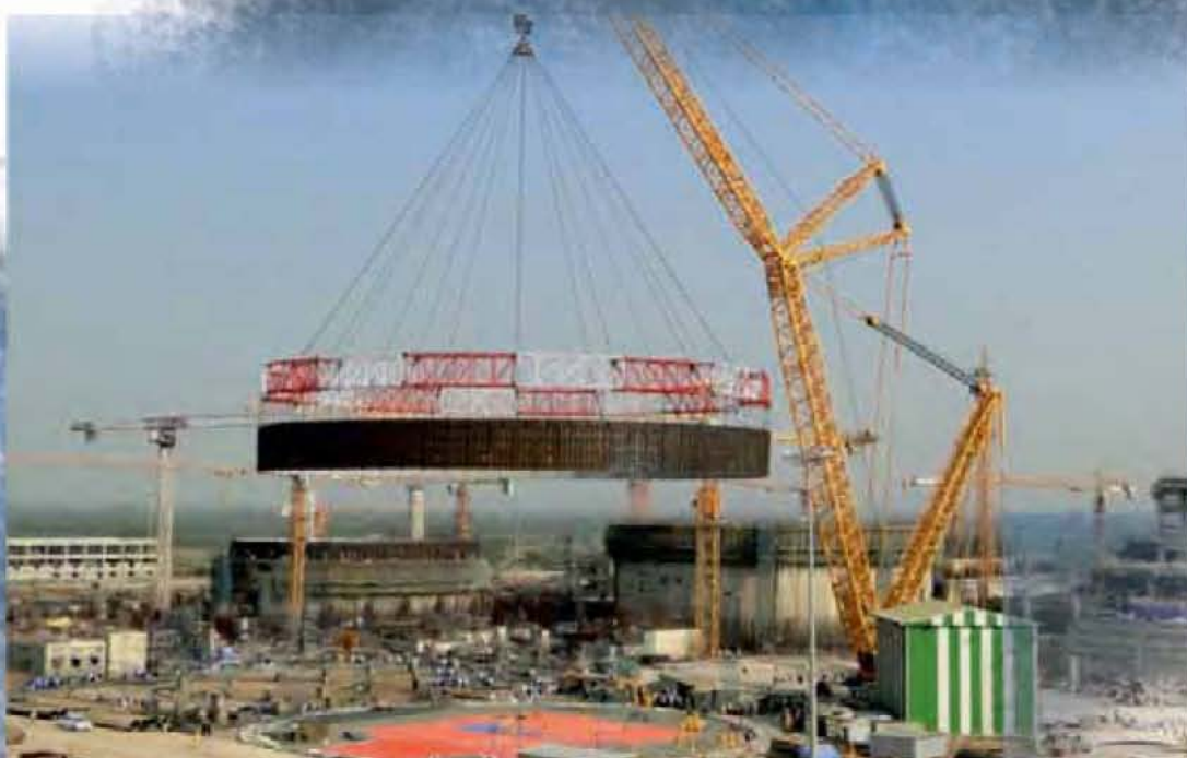
PRL lowering in reactor building in KAPP Unit-3
