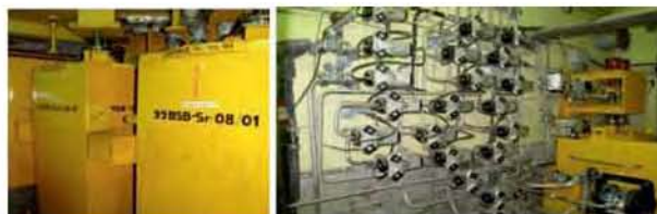
A view of shielded IX- Columns & Valve Station at Pump House for treatment of Historic ILW
