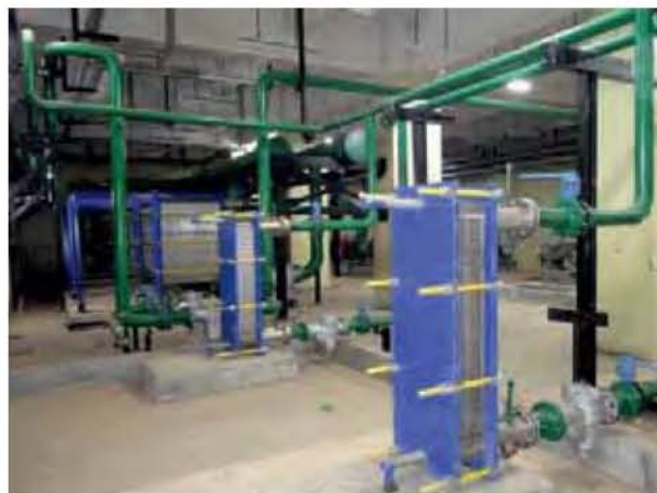
Heat Exchangers & piping
