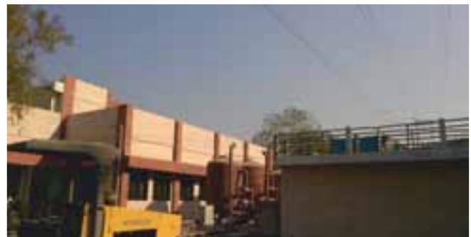
Sewage Treatment Plant at Western Sector in Anushaktinagar is nearing completion
