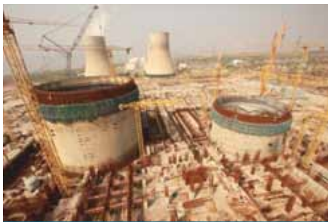
Rajasthan Atomic Power Project -7&8
