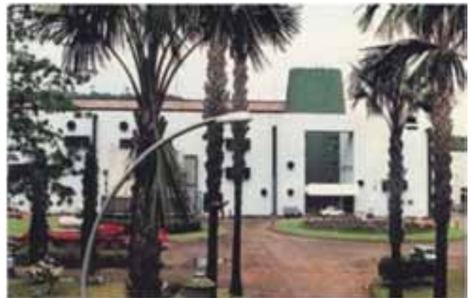
Plutonium Plant, Trombay
