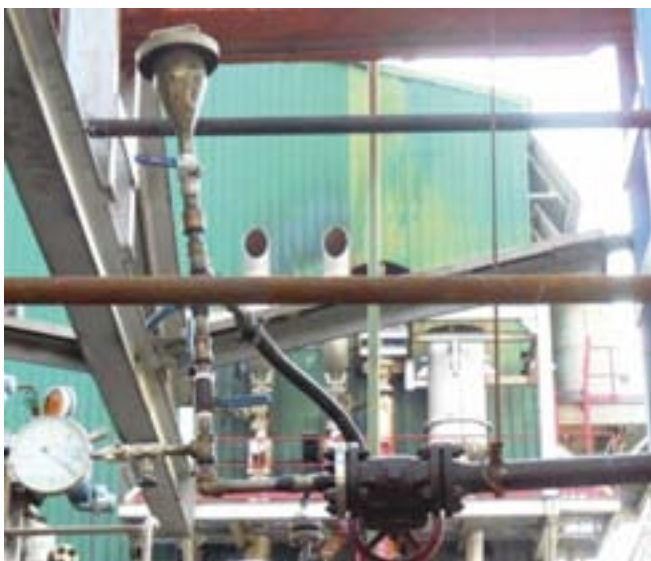
Leak detection study of PET plant, RIL, Dahej, Gujarat
