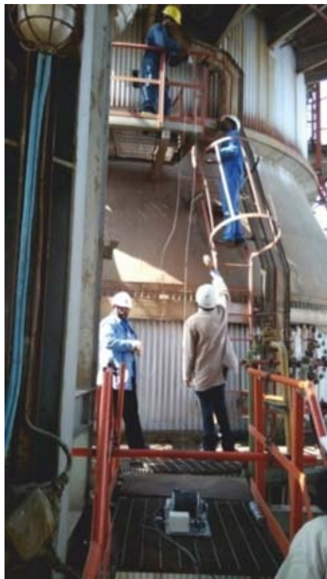
Gamma scanning of Process columns
