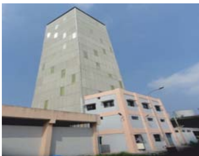
H2O18 Production Plant
