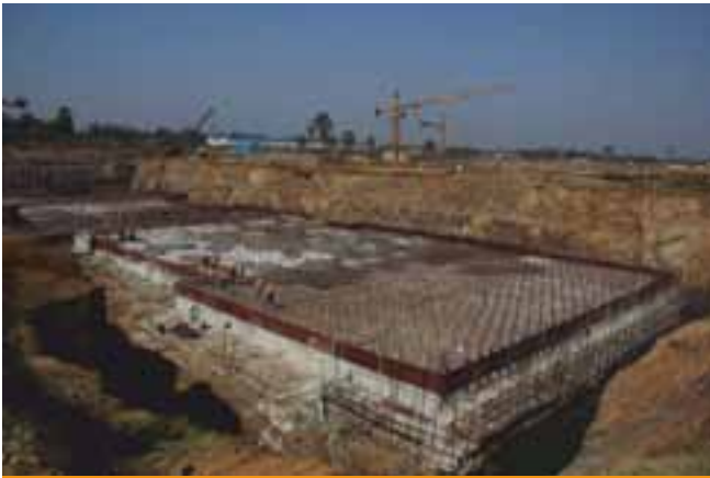
Construction of Raft of one front end block at INRP Tarapur
