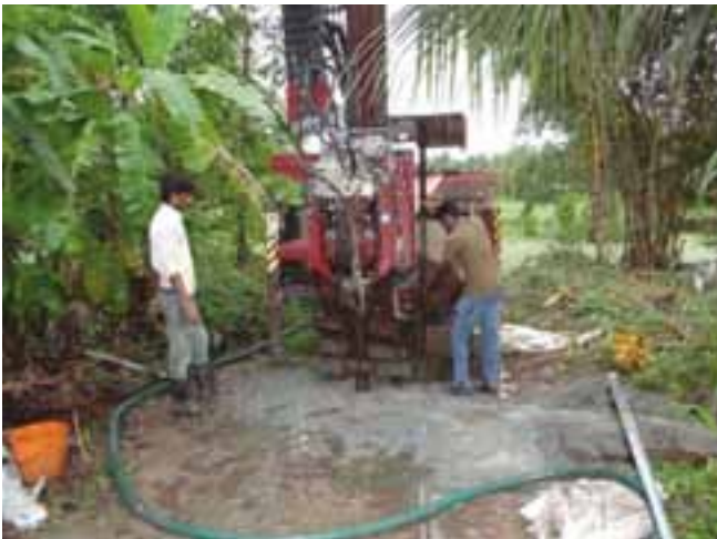
Beach sand drilling operations
