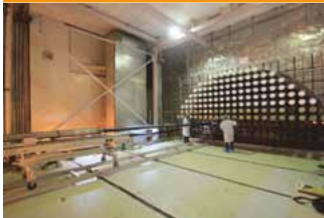
Coolant Channels installation in progress in RAPP-7
