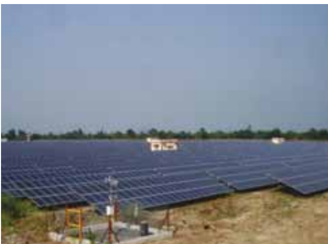
12 MWp Solar P V Cell at Heavy Water Plant, Manuguru
