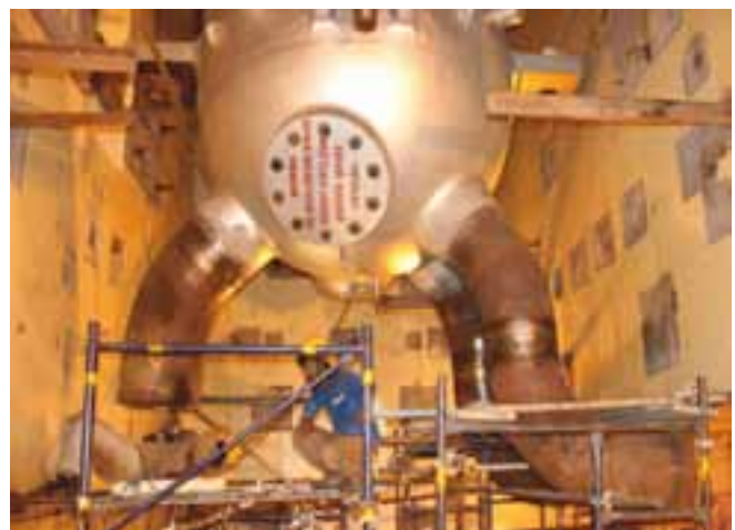
Header-Boiler pipe welding in progress in KAPP-3
