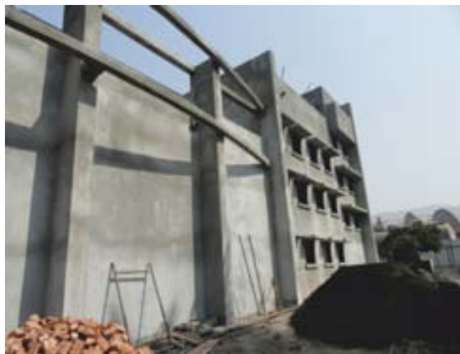
Civil construction for the I-125 seeds plant Facility
