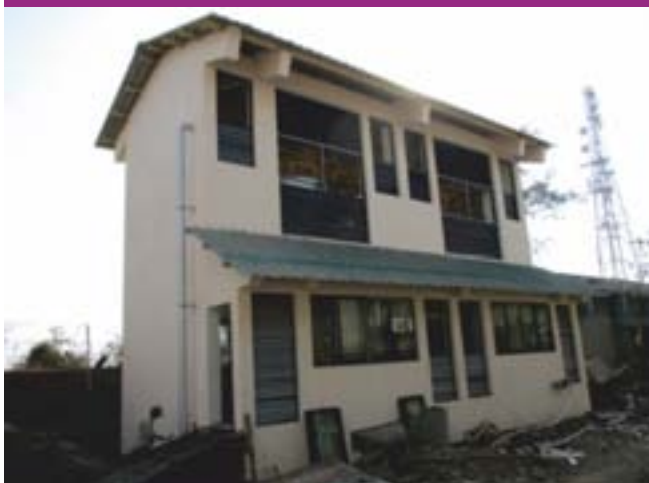
Low level Liquid waste treatment Facility
