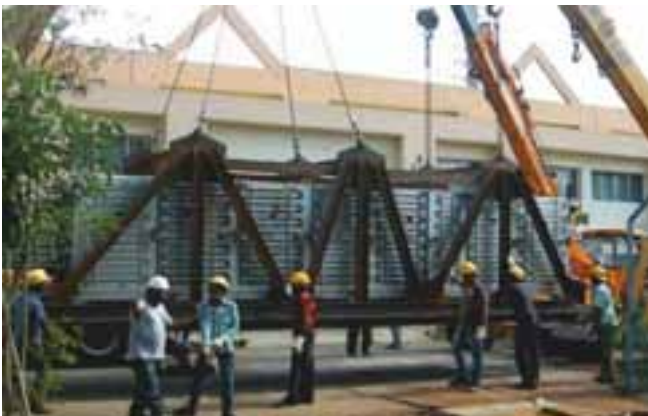
Lifting structure along with the furnace
