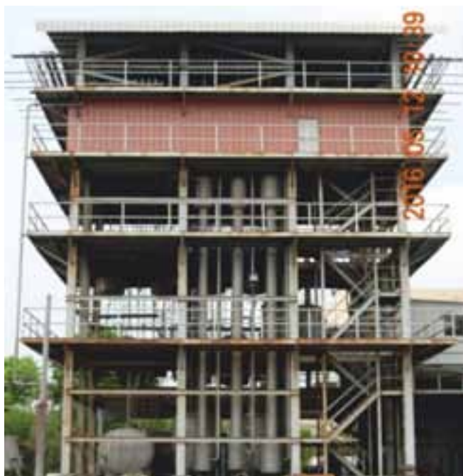
Experimental Facility for Column Testing, Trombay
