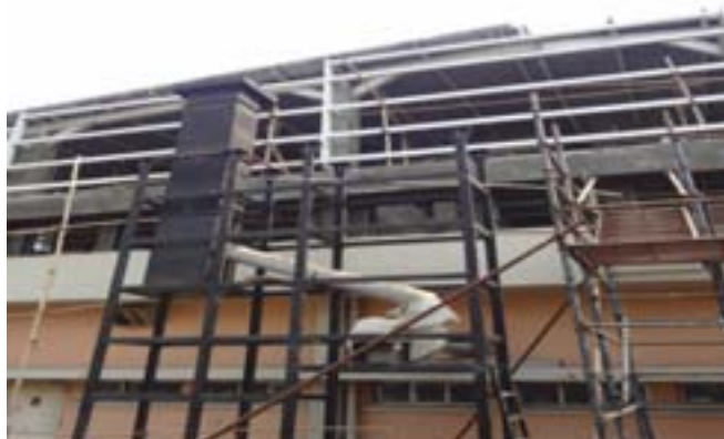
New exhaust system for the fume hoods in synthesis laboratory
