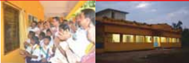
Mid-day meal hall at Kurnipet and School Buildings at Kalache near Kaiga
