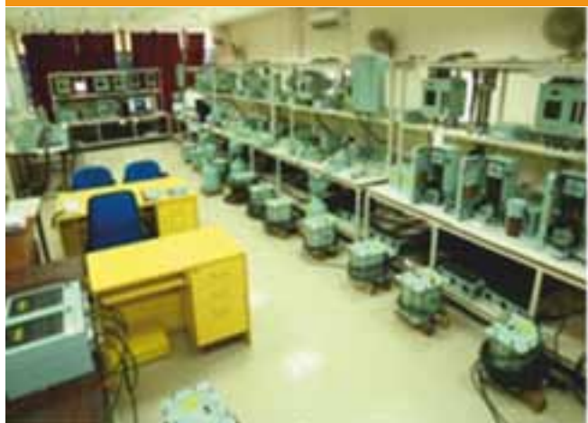
RGMS Units connected at Integrated Test Facility
