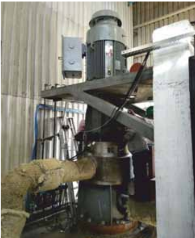
Indigenous 700MWe S/D Cooling Pump in Test Rig
