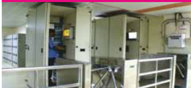
Plastic Scintillator based Portal Monitoring System (PMS)
