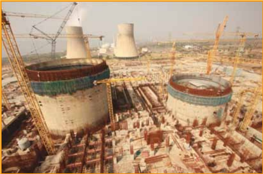
Rajasthan Atomic Power Project - 7&8
