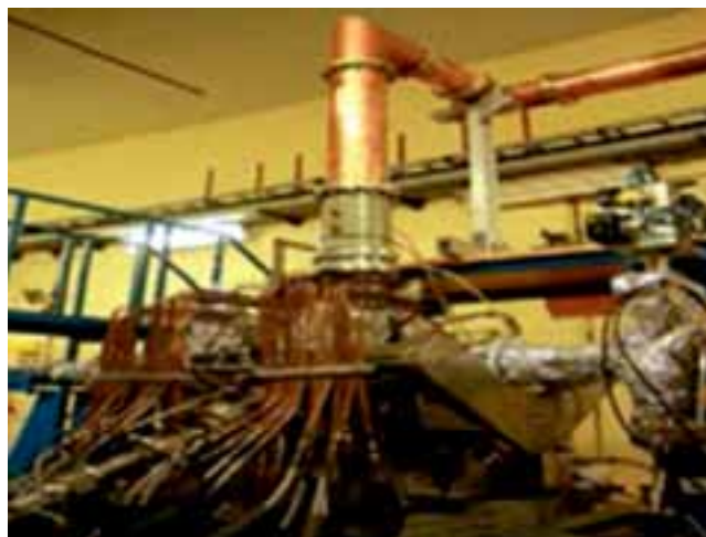
RF Cavity installed and connected to RF power station through transmission line
