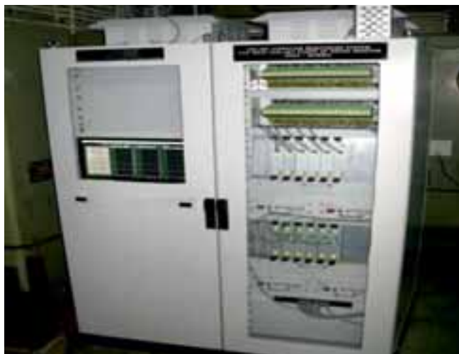
MCPs online vibration monitoring panels
