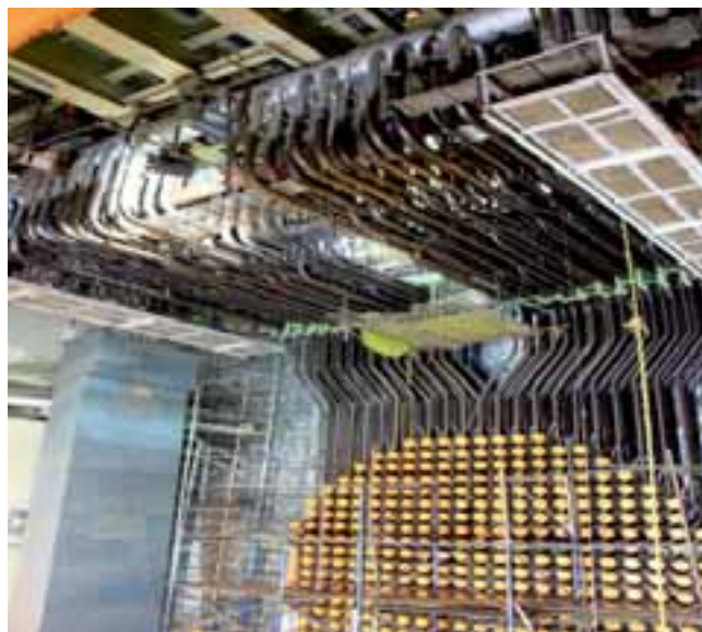
Feeder installation in KAPP-3
