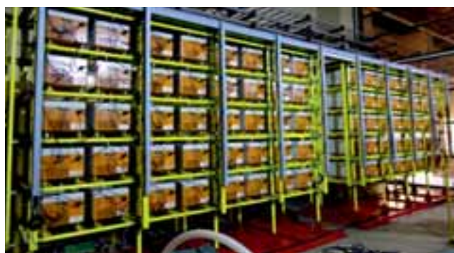
RHVPS with power modules in stacks
