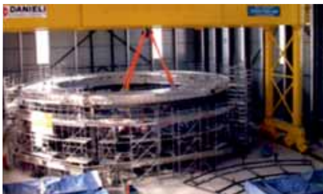
Base Section Tier-1 setup completed and cleared for welding
