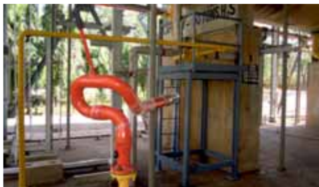
Alkali Spray system for H 2 S tank at HWP, Kota
