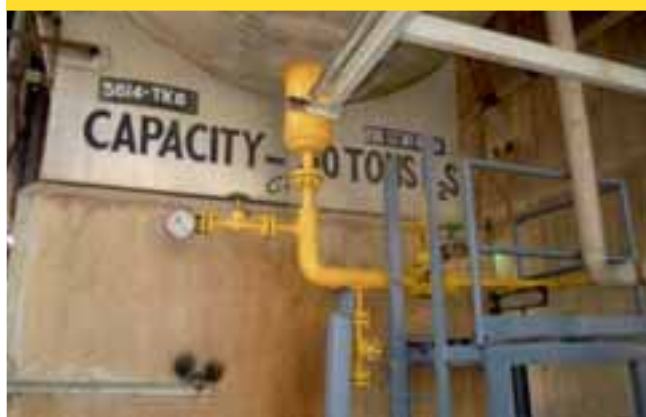
Double Jacketing of drain line and liquid dump line of H 2 S storage tanks at HWP, Kota
