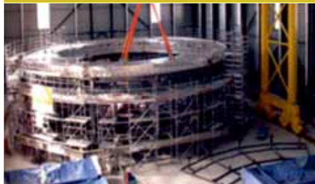
Base Section Tier-1 setup completed and cleared for welding
