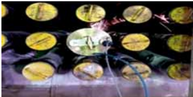
In-situ laser cutting of bellow lip weld joints at KAPS-2 reactor
