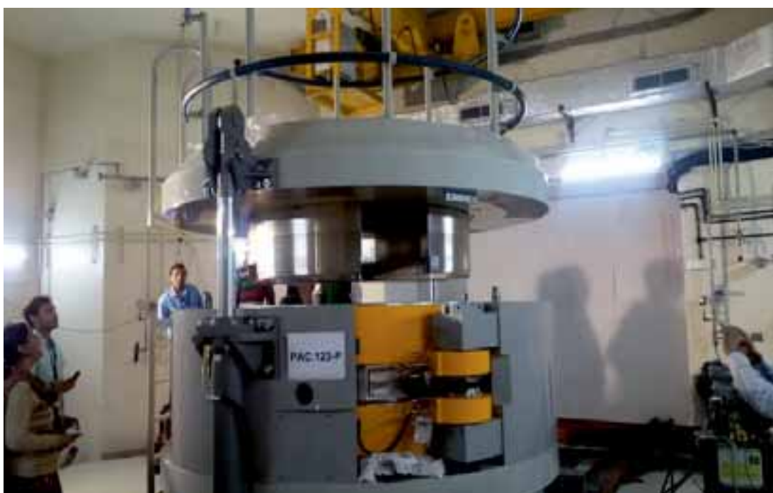
Installation of Medical Cyclotron at VECC
