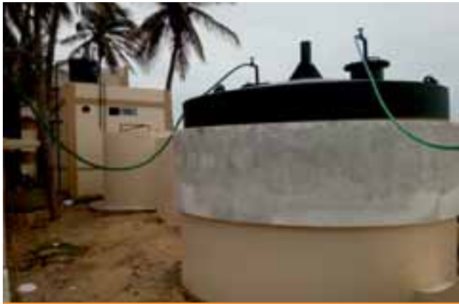
1.0 mt. Per day capacity (Nisargruna) bio-gas plant
