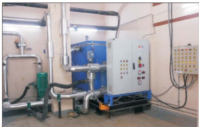
New centralized secondary water pump unit with pipeline and manifold system
