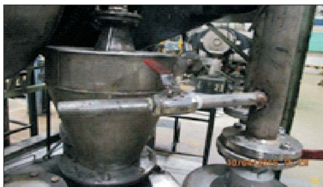
Water flushing provision in the exhaust line of Stabilization Unit
