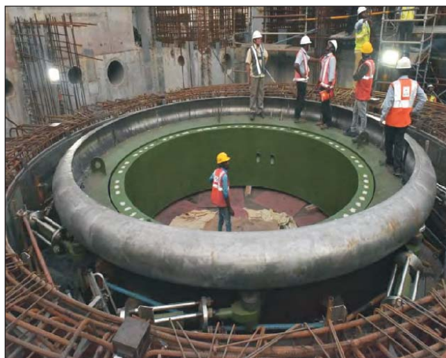
View of Reactor Cavity- Membrane erected -KKNPP-3
