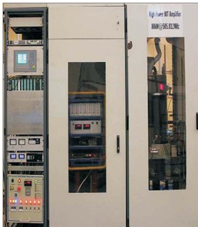
IOT amplifier as set-up in Indus-2
