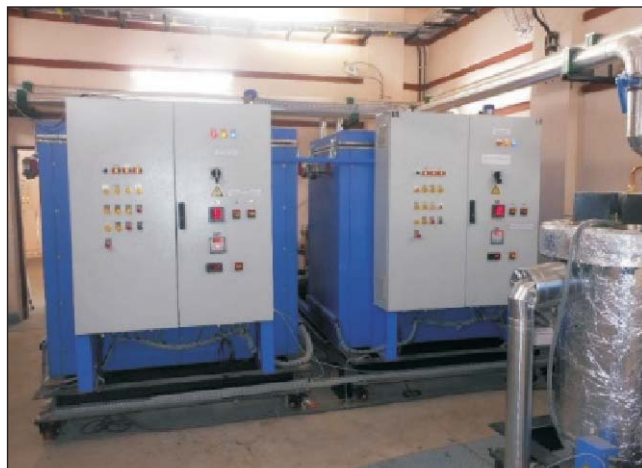
Precision cooling systems installed at newly developed area
