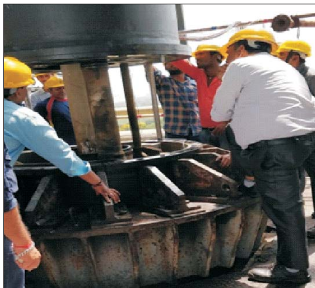
Stage removal of tower 12T2 during MTA at HWP, Hazira
