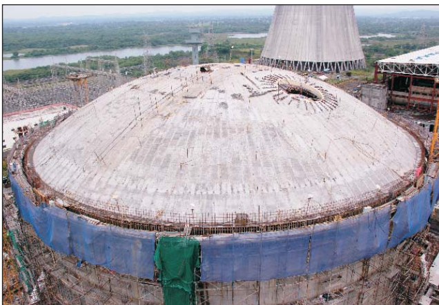
KAPP-4 Reactor Building construction completed with OC
