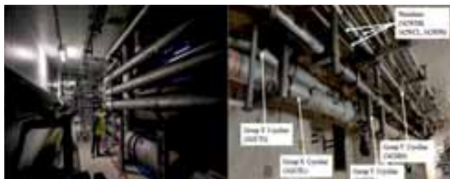
Cryolines and Warmlines manufactured by M/S INOXCVA under installation at ITER site
