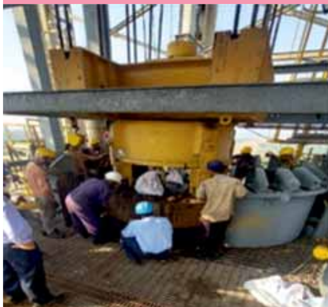
Lifting of individual stage of exchange towers in progress at HWP, Thal
