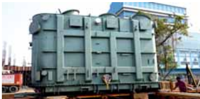
One of the Two 50 MVA Transformers Received at REPS Site, Tarapur
