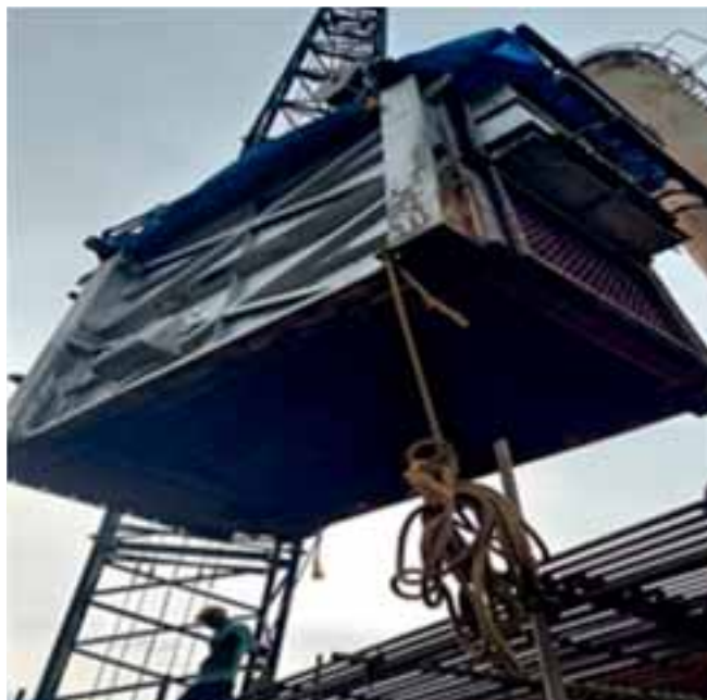
Main Cracker B Super heater replacement in progress at HWP, Thal
