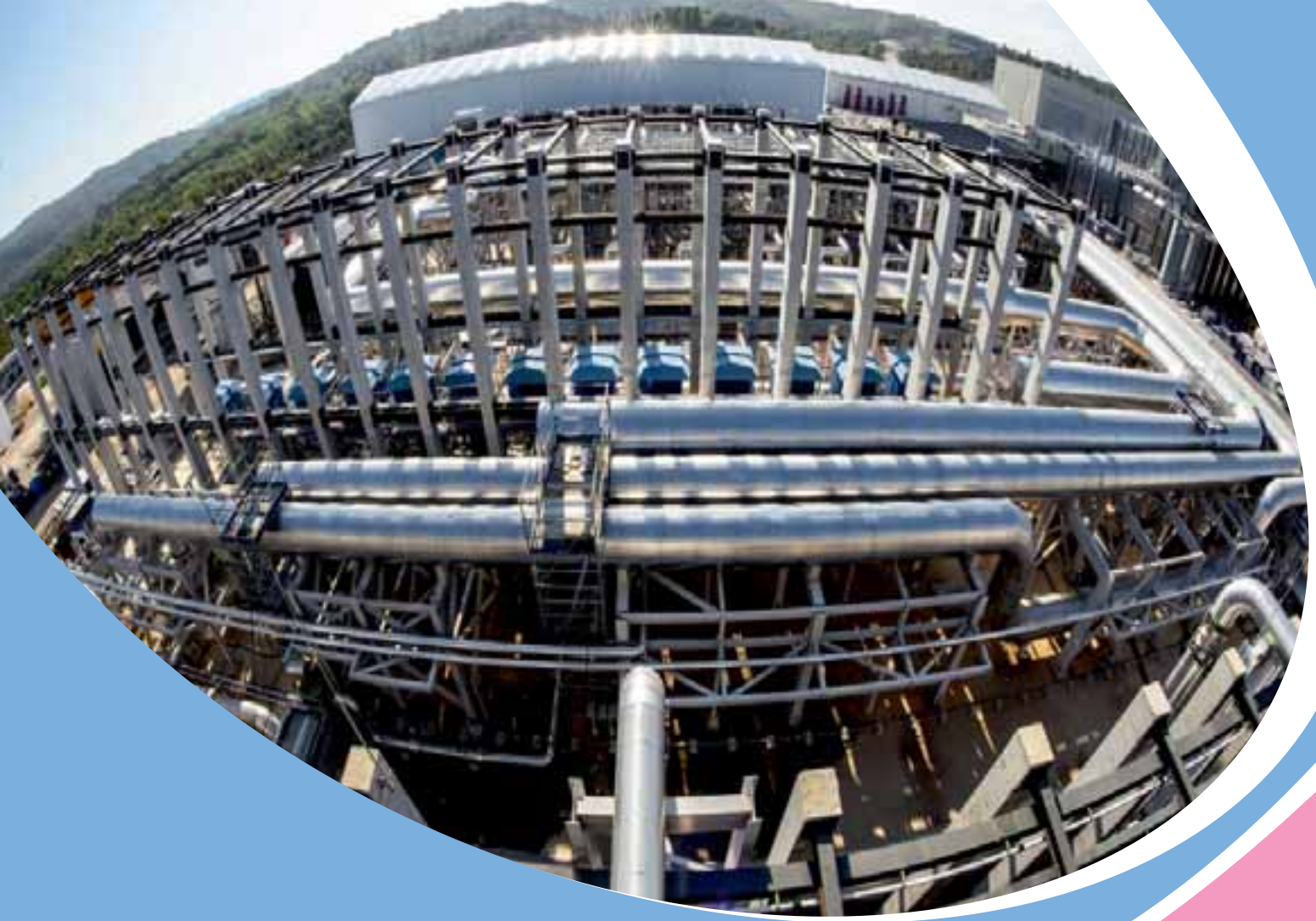
Fish eye view of the cooling water system under installation at ITER site
