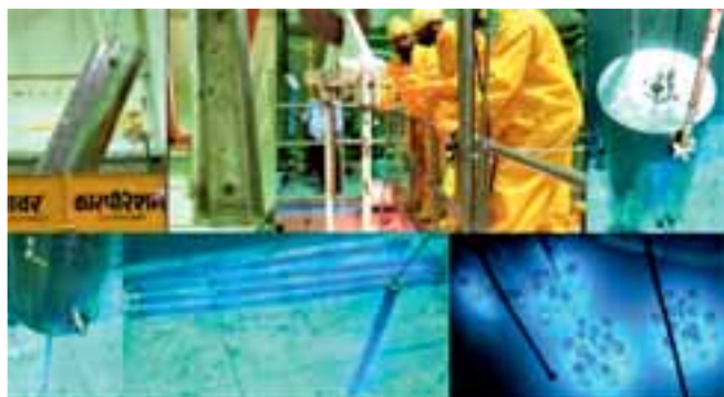
Handling of Cobalt-60 Adjuster rods in BRIT-RAPPCOF storage pool
