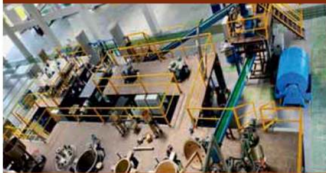
Rare Earth Recovery Plant
