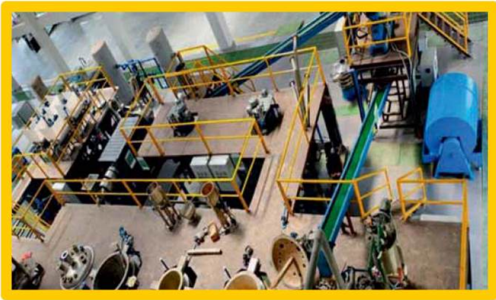
Rare Earth Recovery Plant
