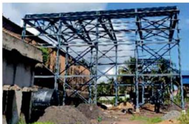
Construction of Module 6-7 (Boiler & scrubber)
