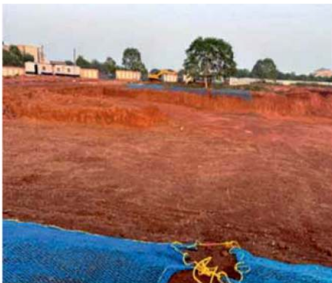
Excavation work at Block-III
