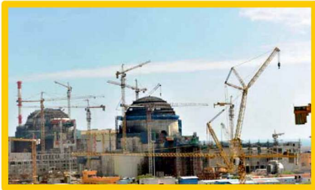
Overall view of Kudankulam Nuclear Power Project (KKNPP) Unit-3&4
